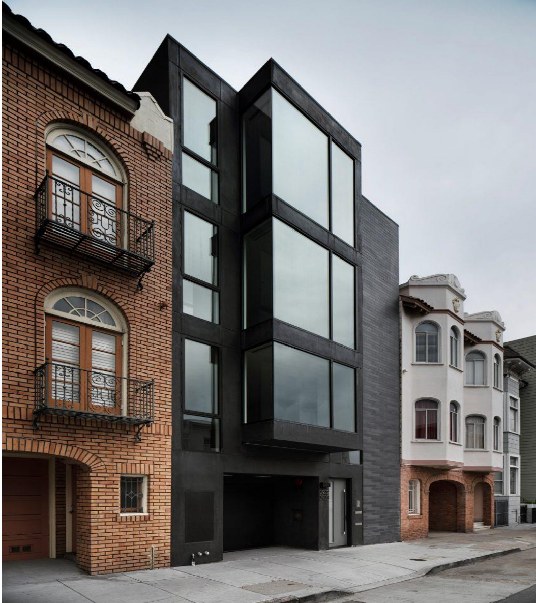
Two styles of full height floor to ceiling multi-story bay windows. Both clearly composing a large percentage of the facades.
