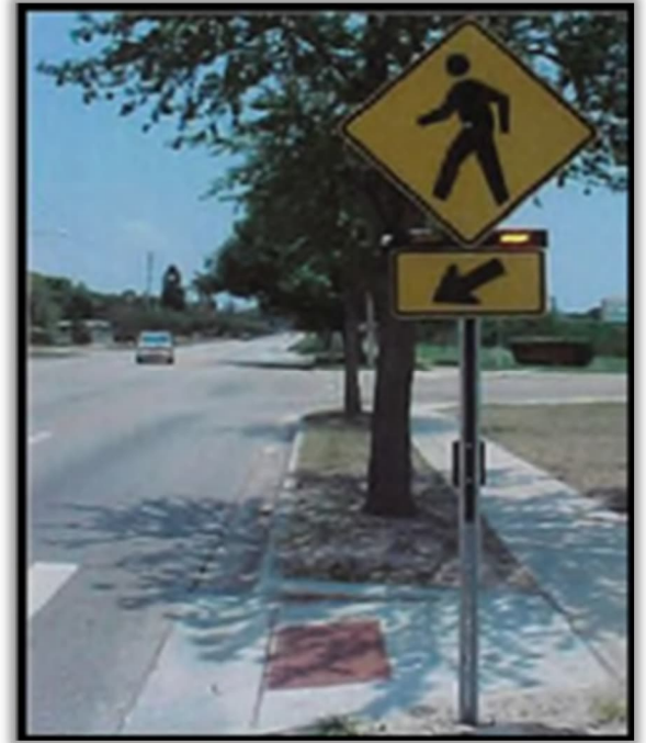
Figure 21 - Mid-block RRFB Crossing Sign
