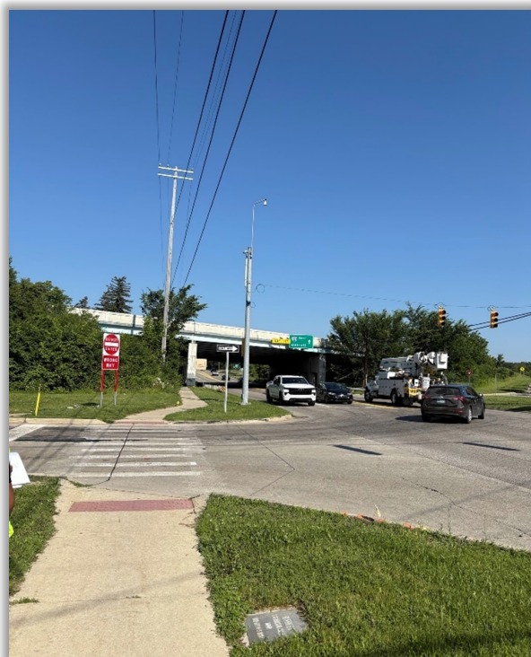
Westbound I-94 Exit Ramp and Jackson Ave Intersection
