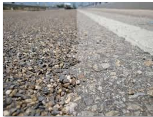
Figure 32 - High Friction Surface Treatment Surface Comparison (Source: FHWA)
