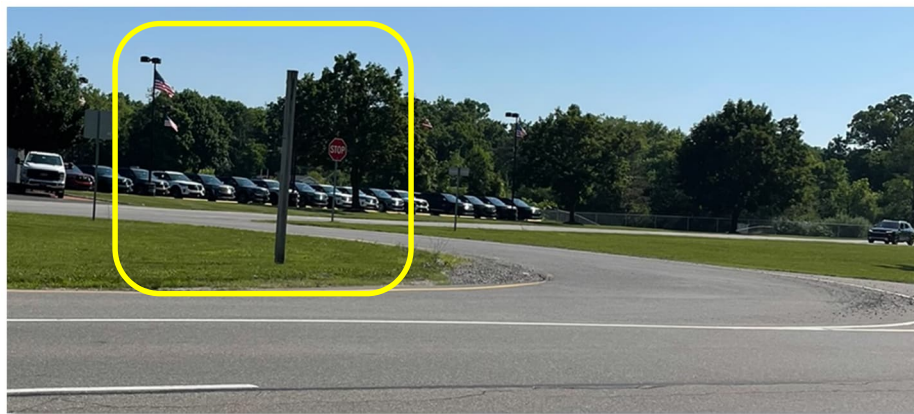
Figure 29 - Eastbound to Westbound Turnaround with Missing Signage
