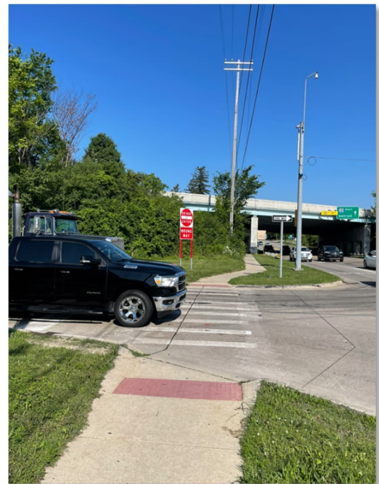
Figure 17 -Westbound I-94 Off-ramp Crosswalk
