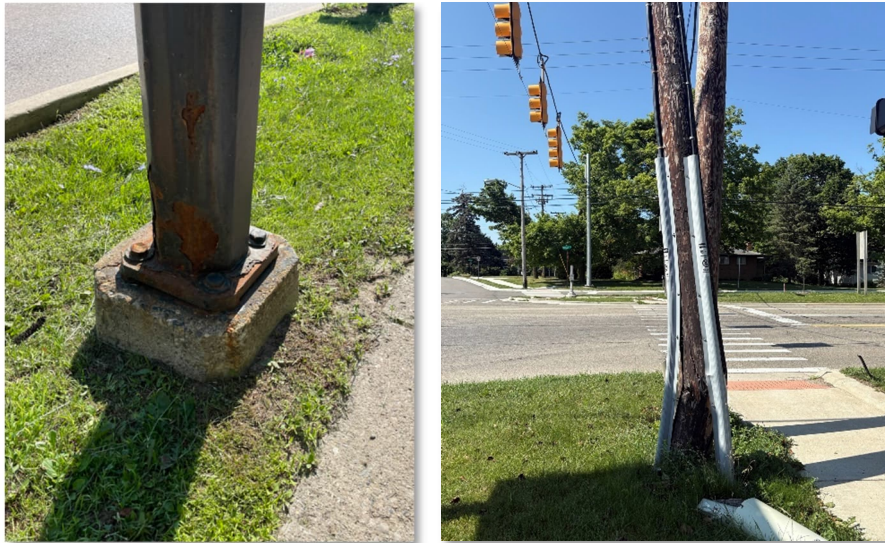
Figure 33 - Observed Pole Foundation Condition
