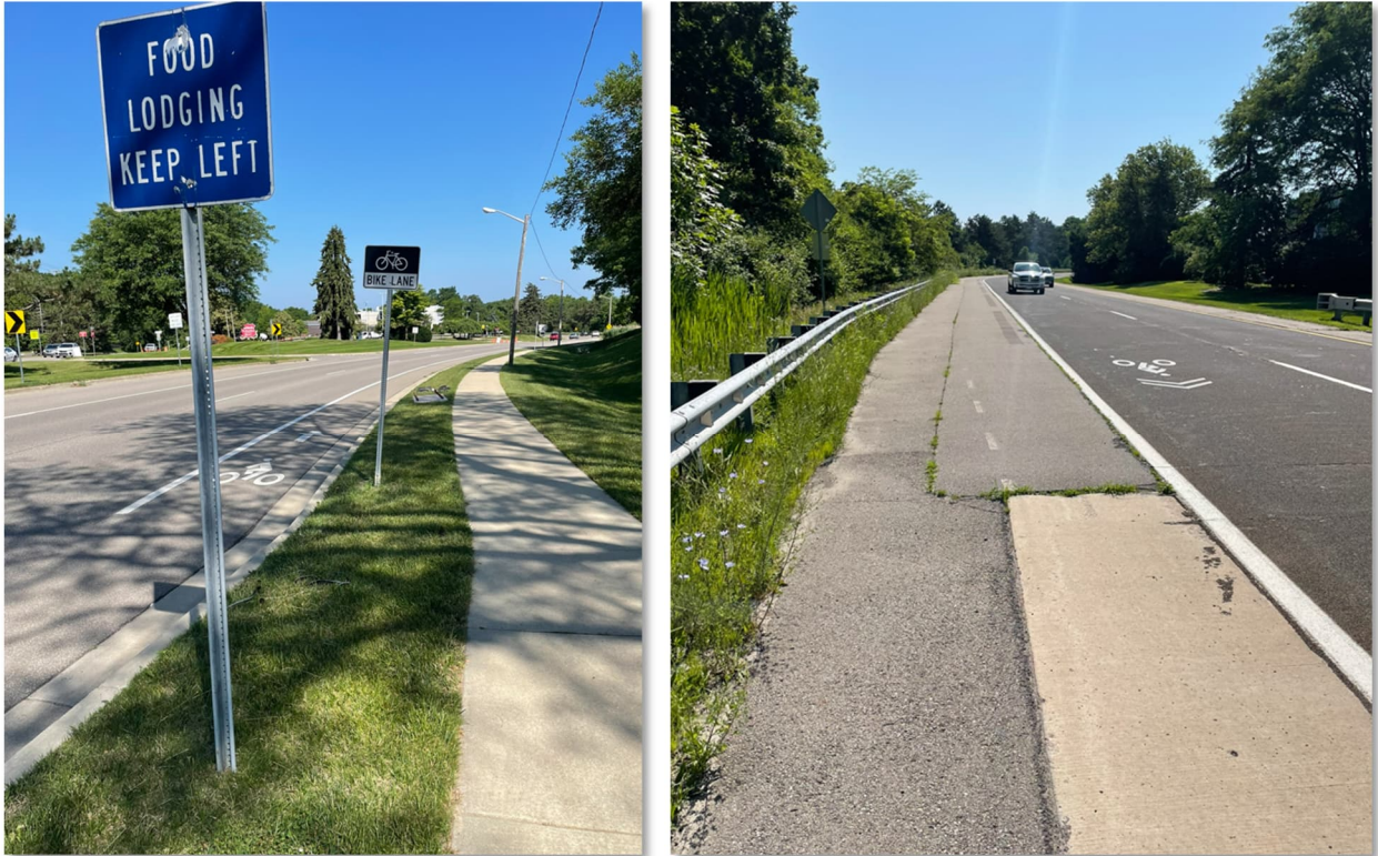
Figure 18 - Westbound Jackson Avenue Bike Lane Signage
