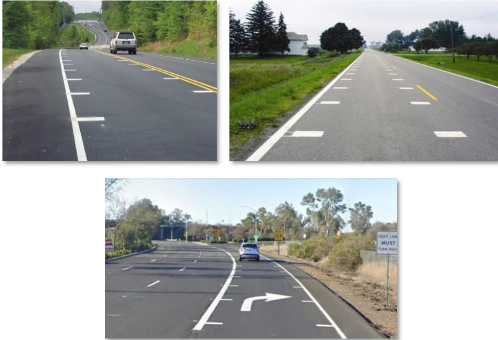
Figure 31 - Optical Speed Bar Examples (Source: FHWA - Top, Caltrans - Bottom)
