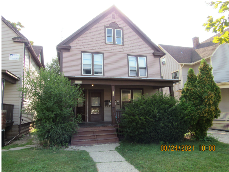
Existing West facade - facing Oakland Ave
