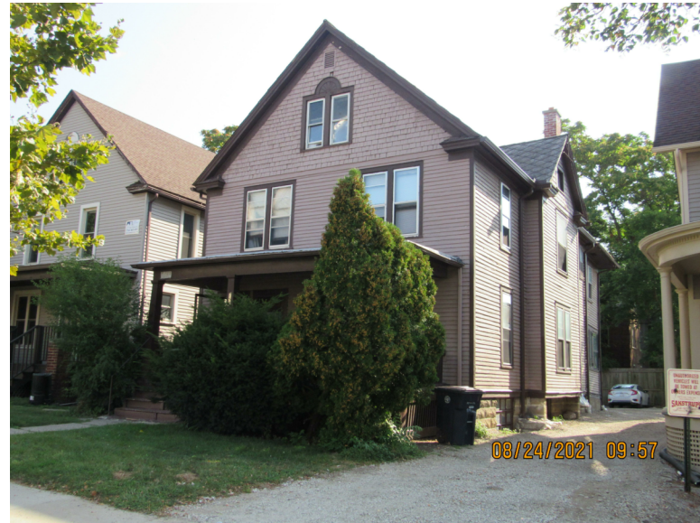
Existing SouthWest facade
