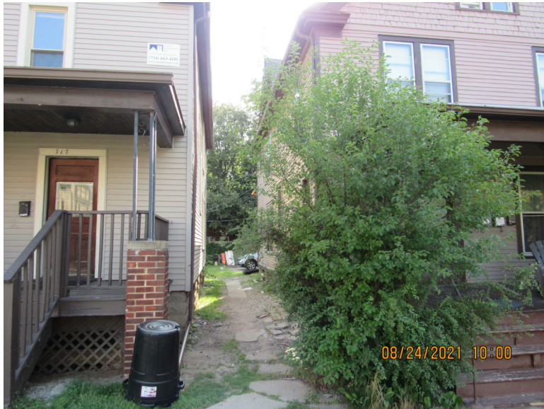
North facade walkway
