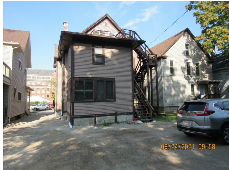
Existing East facade - facing parking
