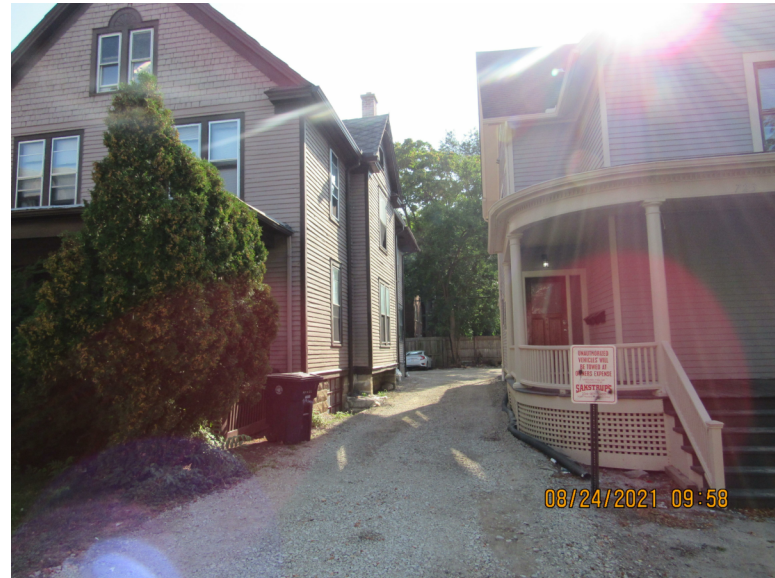
South facade drive aisle
