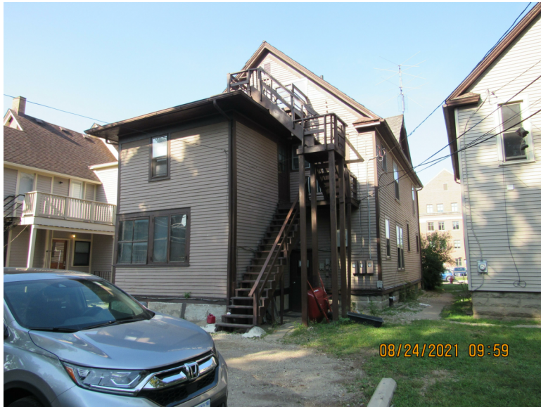
Existing NorthEast facade
