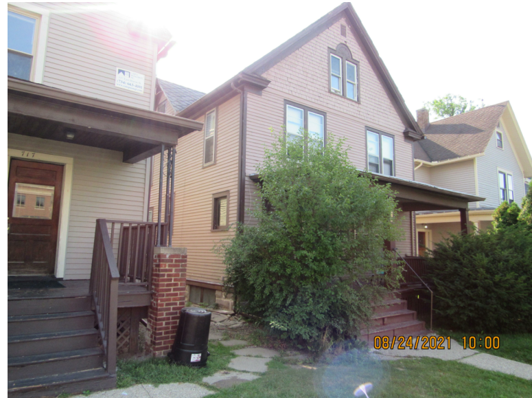
Existing NorthWest facade
