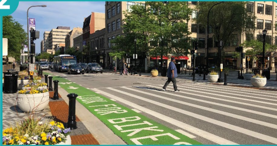
Downtown intersection with bike lane, street furniture, and high visibility pedestrian crosswalk
