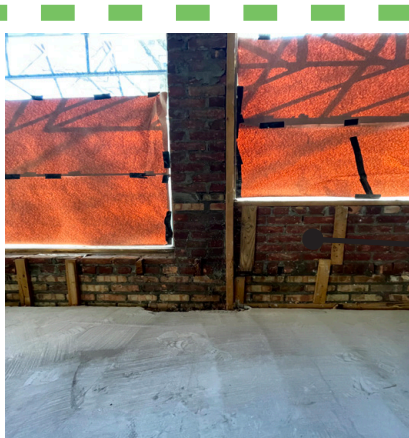
EXISTING GLAZING OPENING WAS REDUCED PREVIOUSLY
