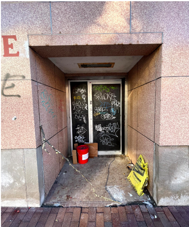
(NORTH) WASHINGTON ENTRY STOREFRONT
