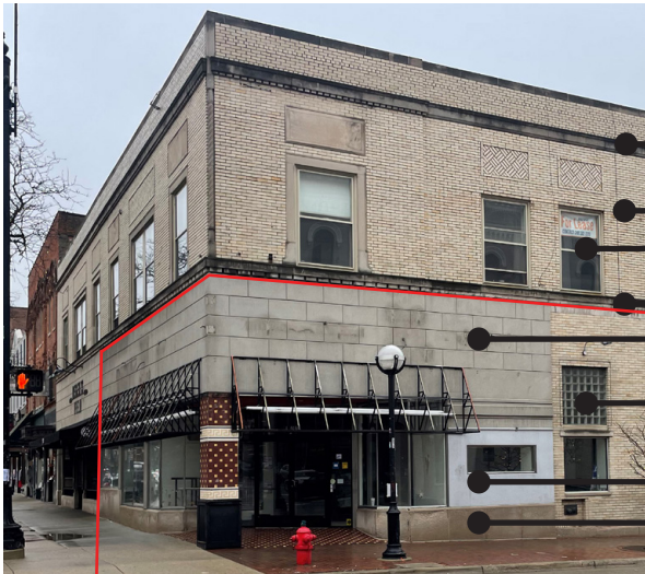
LINE OF SCOPE MAIN / WASHINGTON ENTRANCE
