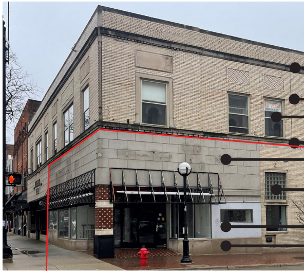
LINE OF SCOPE MAIN / WASHINGTON ENTRANCE
