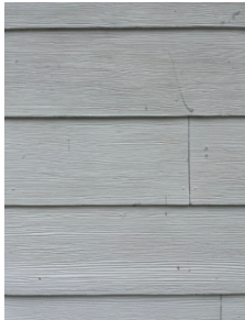
EXISTING 8" HORIZONTAL TEXTURED CEMENT BOARD SIDING, PAINTED
