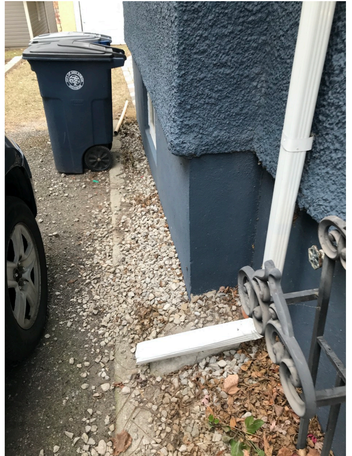
EXISTING: STUCCO FINISH
