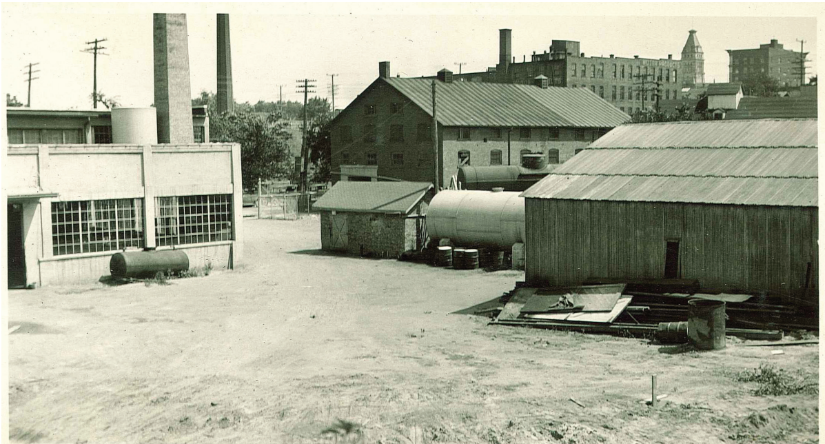
Undated late 1920's photo of yard with the bean warehouse in the background purchased from Michigan Milling. This building, which was used to store trucks and road tar, was torn down prior to 1934 when the rail trestle was built by the CWA. It is probable that the brick in this building was used to build the CWA garage shown in the photo below.
