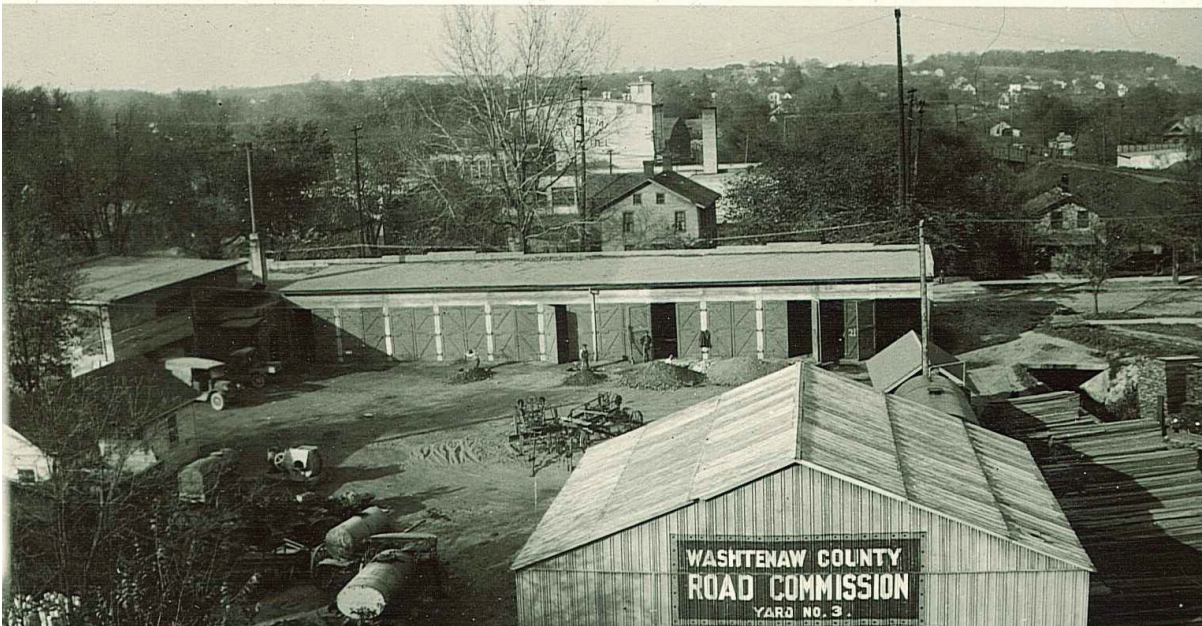
October 1924 photo showing laborers digging footings for the new steel framed high bay space behind the earlier 12 bay "private garage."
