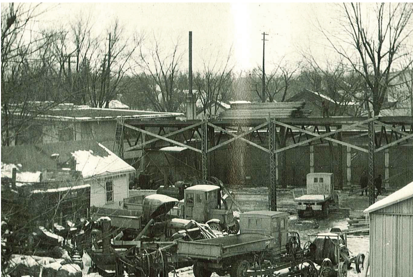
Photo showing construction of the steel framed high bay space January 10, 1925.
