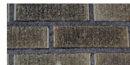
Buff "rug faced" brick on pilasters.
