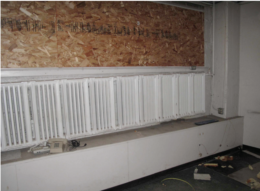
Picture M3: Existing radiators to be demolished
