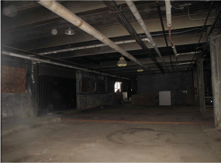
Picture M2: Existing piping to be demolished
