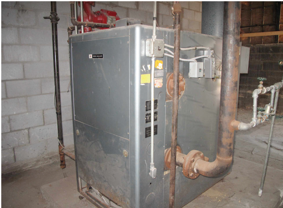
Picture M1: Existing boiler to be demolished
