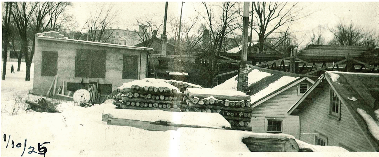
January 10, 1925 photo of the concrete machine shop built between 1916 and 1925. Portions of the lower floor appear to have been incorporated into the 1928 addition. The southern lower wall and parts of the east lower wall are still visible within the building today. The ad hoc column spacing and complex structural systems in this part of the building were the result of needing to build around these existing structures. These structures were later demolished and a new concrete two-story building was threaded through the remaining open space.
