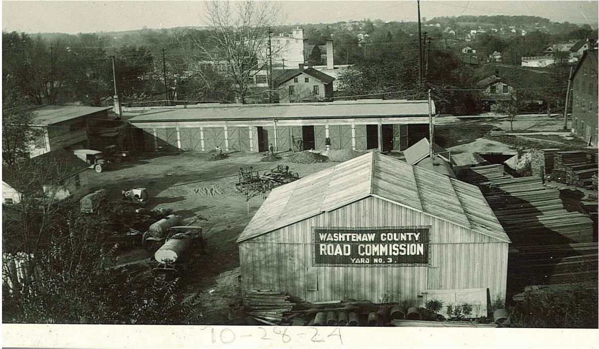
October 28, 1924 photo showing the existing 12 bay "old garage" building at the top of the picture with the two story concrete machine shop on the left. Four laborers are shown in front of the garage digging footings for the new high bay garage.
