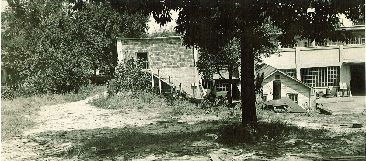
1928 photo of site showing the existing machine shop and second story office with temporary structural clay-tile infill which will be removed when new addition is built. Portions of the first floor "old concrete machine shop" appear to have been incorporated into the new 1928 addition. The small gap between the two buildings just to the left of the tree trunk is probably the remains of the earlier cooper shop. Excavation for the new addition will start soon as the steam shovel visible to the right of the tree trunk has just arrived on site.
