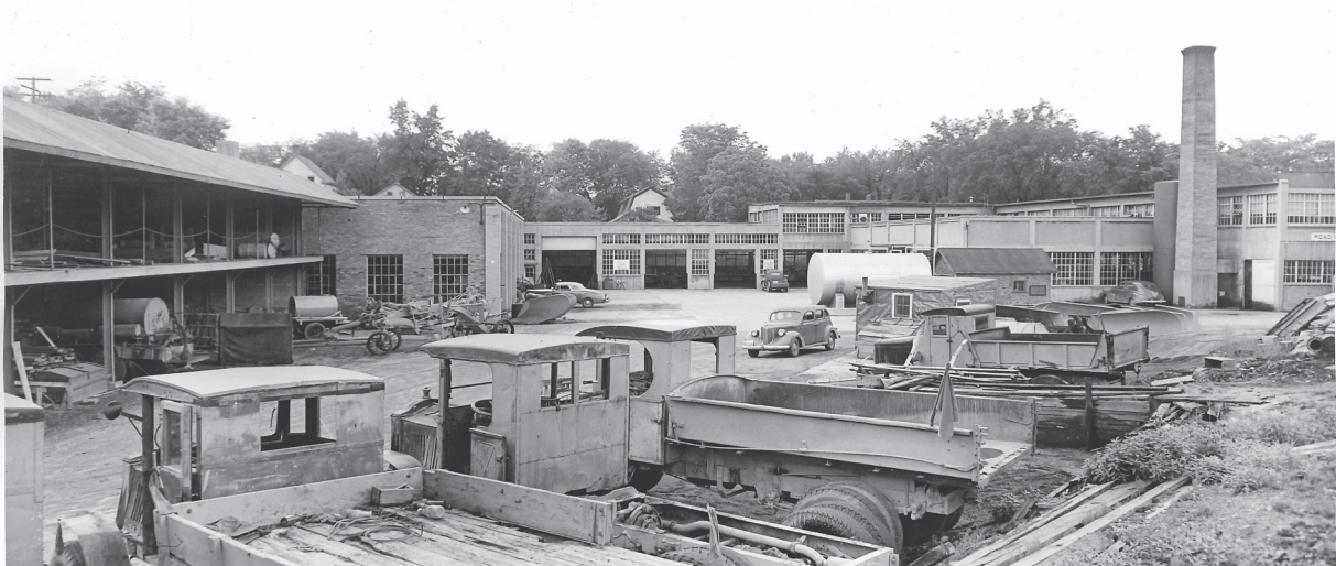
June 1940 panorama photo showing the entire yard with the 1934 CWA Welfare additions on the left, the 1928 machine shop in the center and two-story office and garage building on the right. Early 1920's era dump trucks are "retired" along the Ann Arbor Railroad grade where the spur to the trestle dump is located. Little has changed from the date of this photo to the present time. The large fuel oil tank next to the brick boiler flue and the 15,000 gallon gasoline tank with its adjacent brick pump house has been removed.
