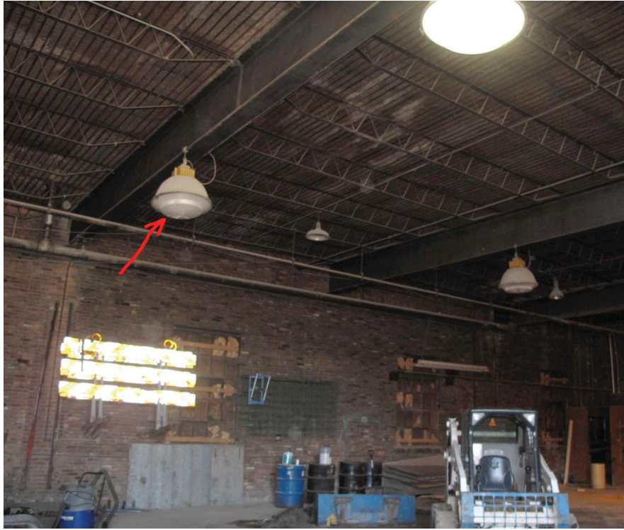
Picture E3: Existing lighting Condition Evaluation
