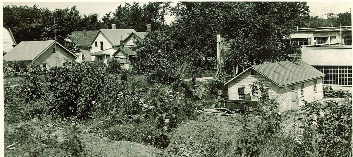
1928 photo of a Bucyrus Erie steam-shovel excavating a portion of the hill behind to make way for the 1928 new office and machine shop addition. The huge extent of this excavation can be seen by standing at the north end of the existing car wash property at 318 West Liberty and looking down at the 1934 CWA storage building. Approximately sixteen to eighteen feet of earth was removed from the south end of the Road Commission Property.
