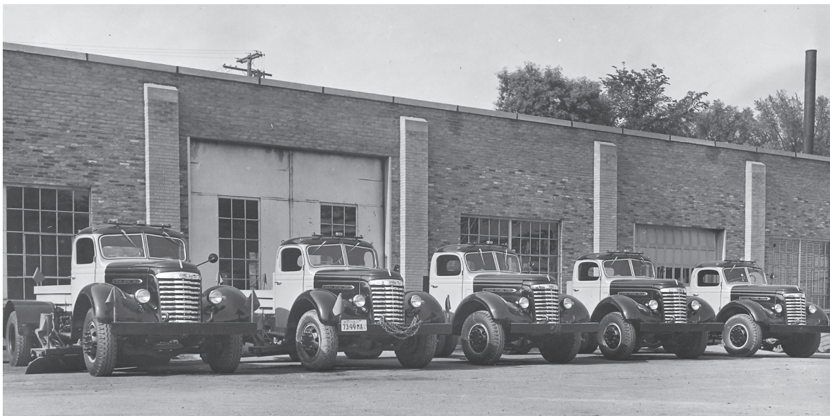
June 4, 1940 photo of the 1934 CWA Welfare Garage with five new GMC snowplow and utility trucks. The brick used for the lower 2/3 of the walls is reclaimed. It is possibly from the two-story bean warehouse on the site which had been recently demolished. The upper third is new brick. The "rug-brick" cream colored pilasters are also new brick.
