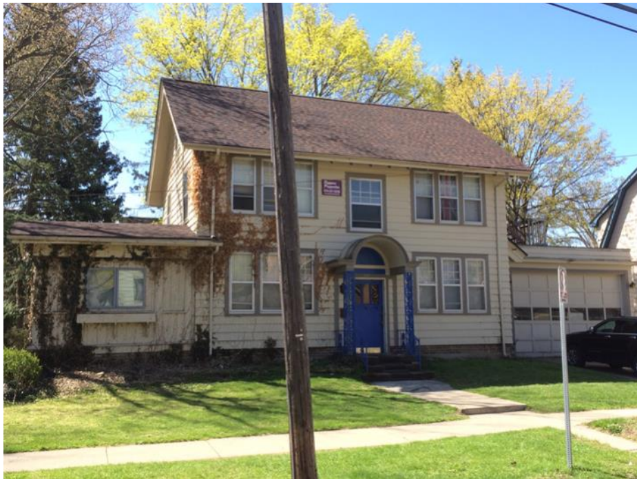
722 McKinley (across street - south)
