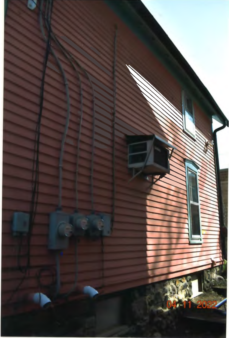
South Elevation next to 533 Eliz
