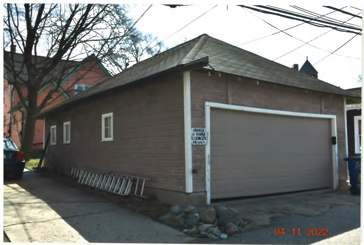
Old 4Four Car Taxi Garage NW Corner - On Alley
