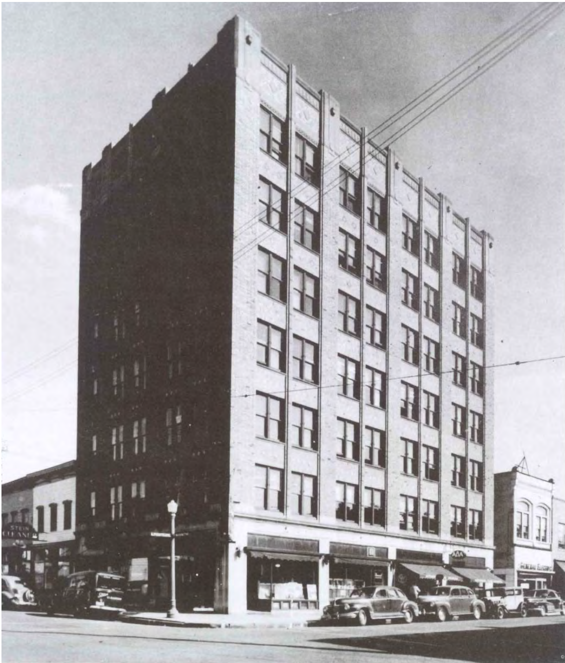
Undated photo of the northwest corner of the building, circa 1950 based on the cars. Note the small windows above the transom, and the four storefronts on S. Fourth. By the time this photo was taken, the corner tenant space and its four openings had been modified. Although taken after the period of significance, this photo illustrates how much of the original fabric remained by c. 1950, and can be compared to extant materials in place today.
