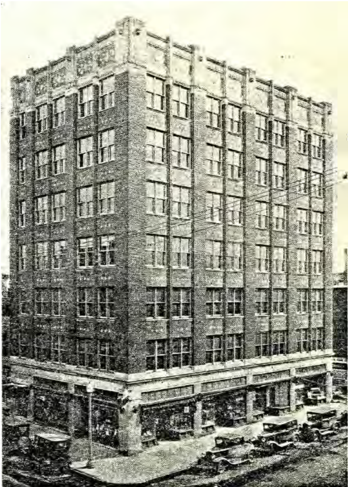
Undated photo of the northwest corner of the building, circa 1930 based on the cars, and similar to the colored rendering of the building from the same time. Note the small windows above the transom, and the four storefronts on S. Fourth, all having the same configuration.
