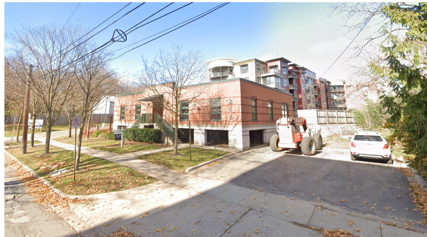
214 W. Kingsley SE Street View
