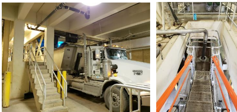
Figure 20: Biosolids Cake Truck Loading. (Left: Open Bed Biosolids Cake Truck loading during Winter, Right: Liquid Biosolids Sealed Tanker Truck loading in Summer)
