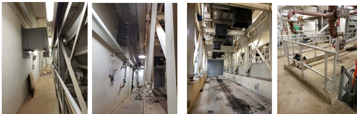
FIGURE 10: TRUCK LOADOUT HOPPERS AND TRUCK BAY
