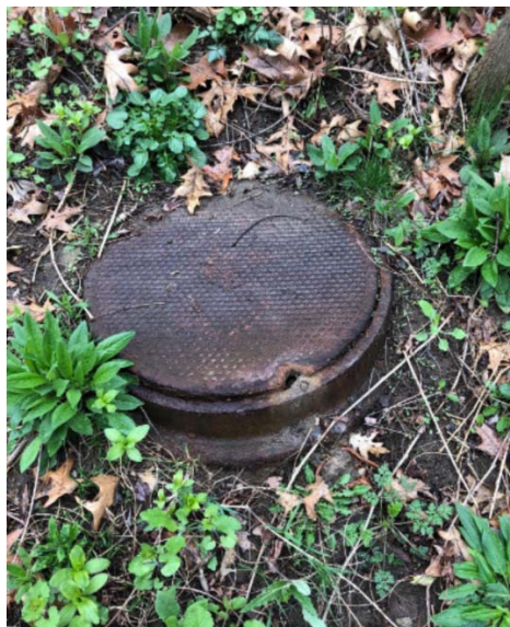
FIGURE 17: OLD DIXBORO MANHOLE #71-61488
