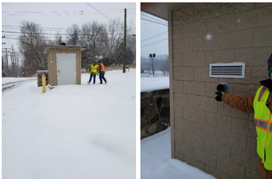
FIGURE 15: VENT VAULT
