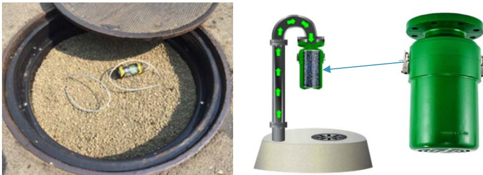
Figure 6-3. Manhole based odor control: “Peacemaker” style manhole insert (left), Goose neck external carbon canister (right)
