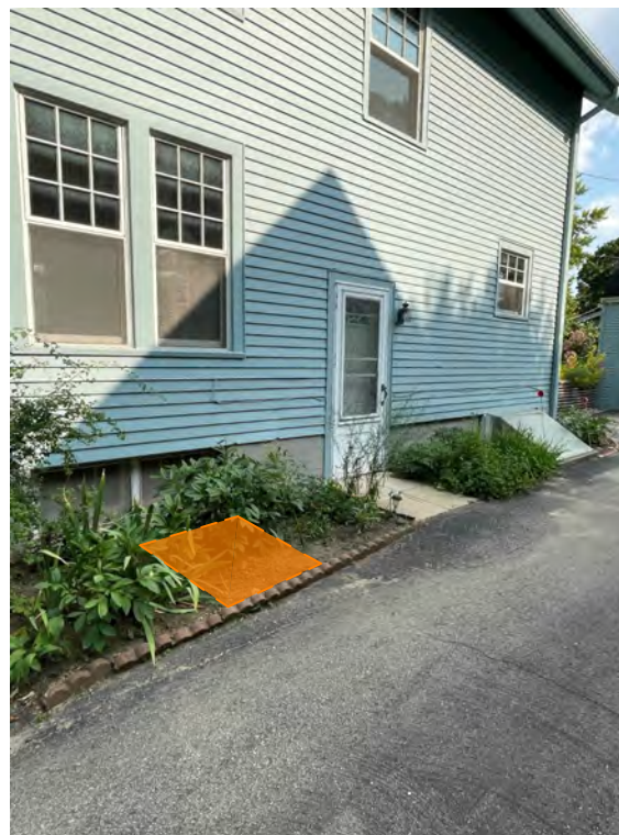
NEW WINDOW WELL ALONG WEST SIDE OF HOME
