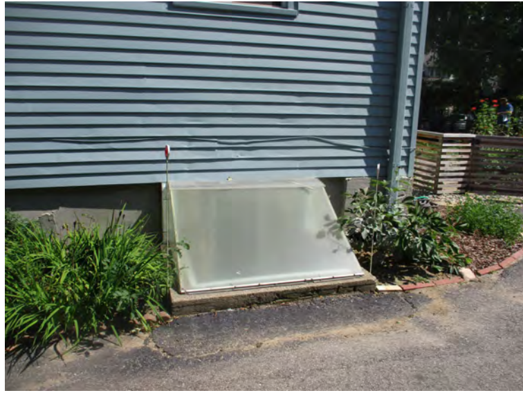
EXISTING WINDOW WELL NEAR SOUTHWEST CORNER OF HOME TO BE INFILLED
