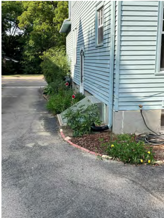
EXISTING WINDOW WELL NEAR SOUTHWEST CORNER OF HOME TO BE INFILLED
