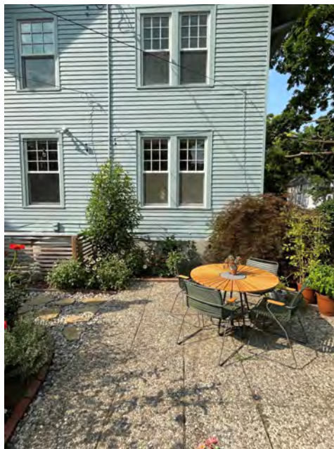
DOUBLE WINDOW ARRANGEMENT TO BE REMOVED FOR NEW DOOR WITH NEW LANDING AND STAIRS DOWN TO PATIO
