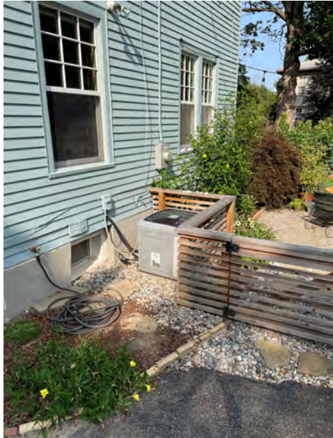
A/C UNIT TO BE RELOCATED
