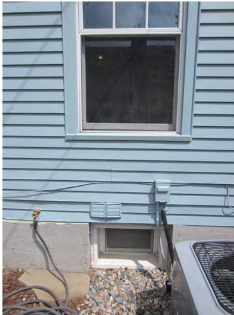
WINDOW & BASEMENT WINDOW TO BE REMOVED
