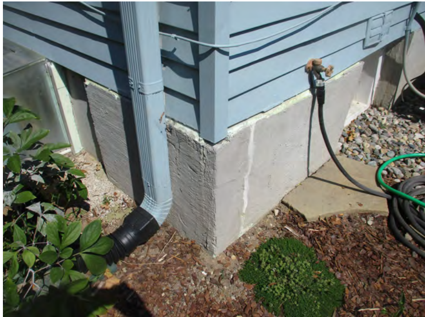
SOUTHWEST CORNER OF EXISTING HOME TO REMAIN
