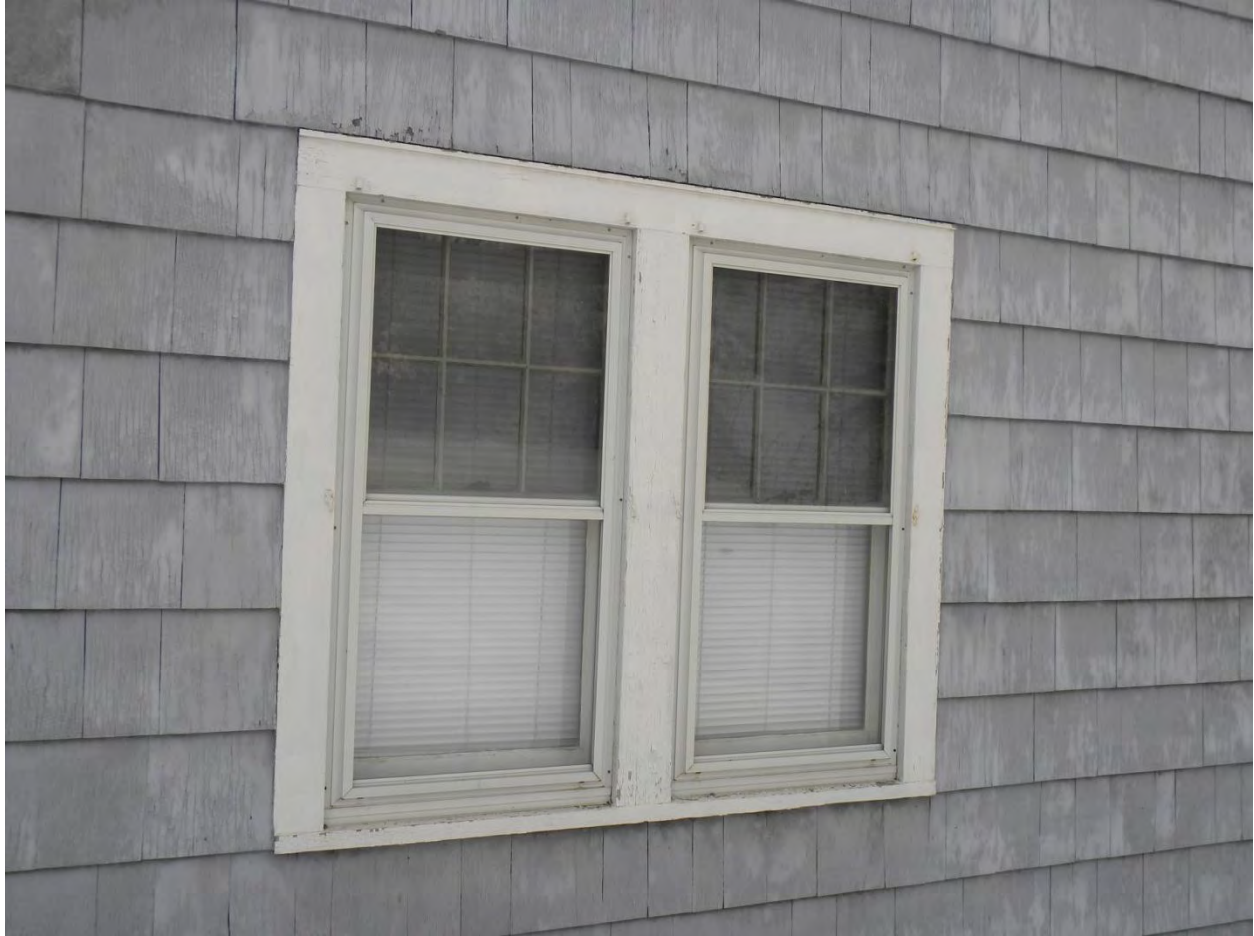
Existing windows with trim boards and aluminum storm windows
