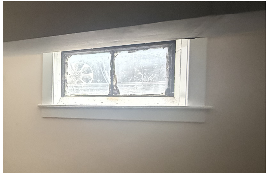
PHOTOS OF EXISTING CONDITIONS MULTIPLE PHOTOS OF EXTERIOR AND EXISTING WINDOWS
