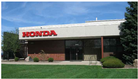
EXISTING BUILDING EAST
