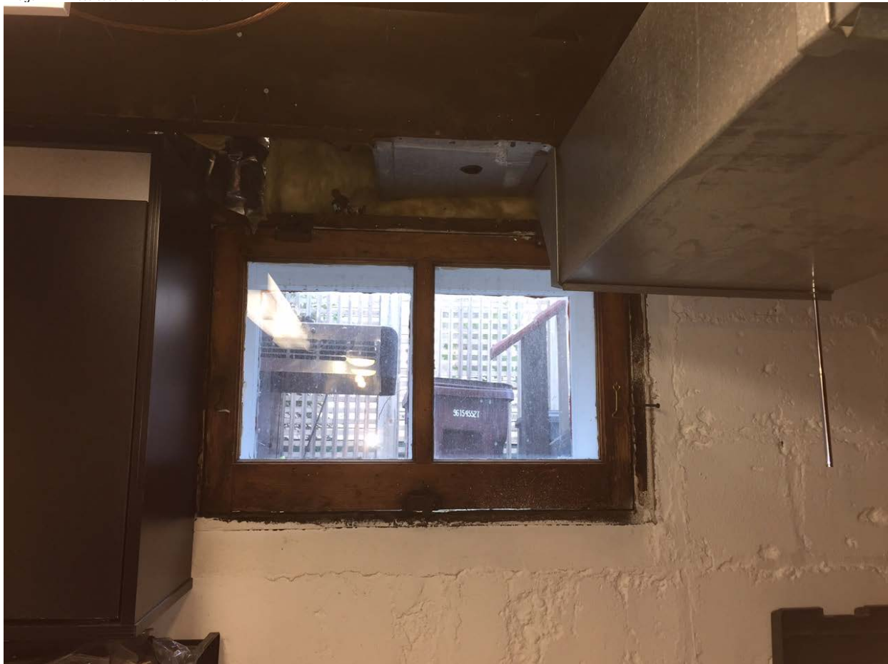
Image #1 - West basement window interior view
