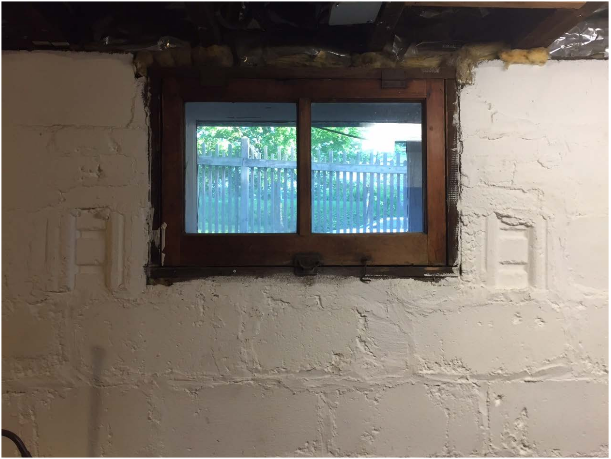
Image #6 - South basement window exterior view
