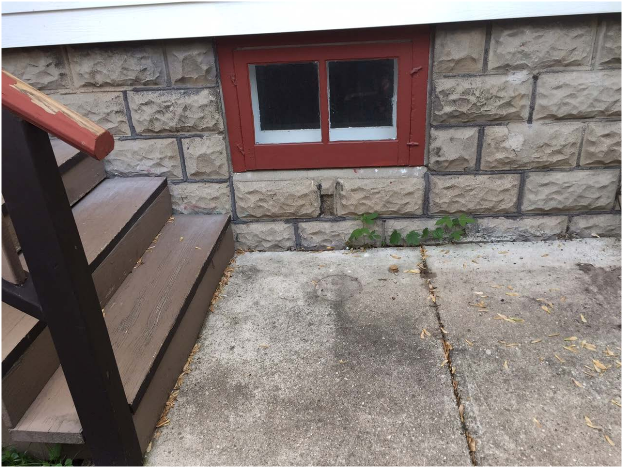
Image #4 - West basement window exterior view
