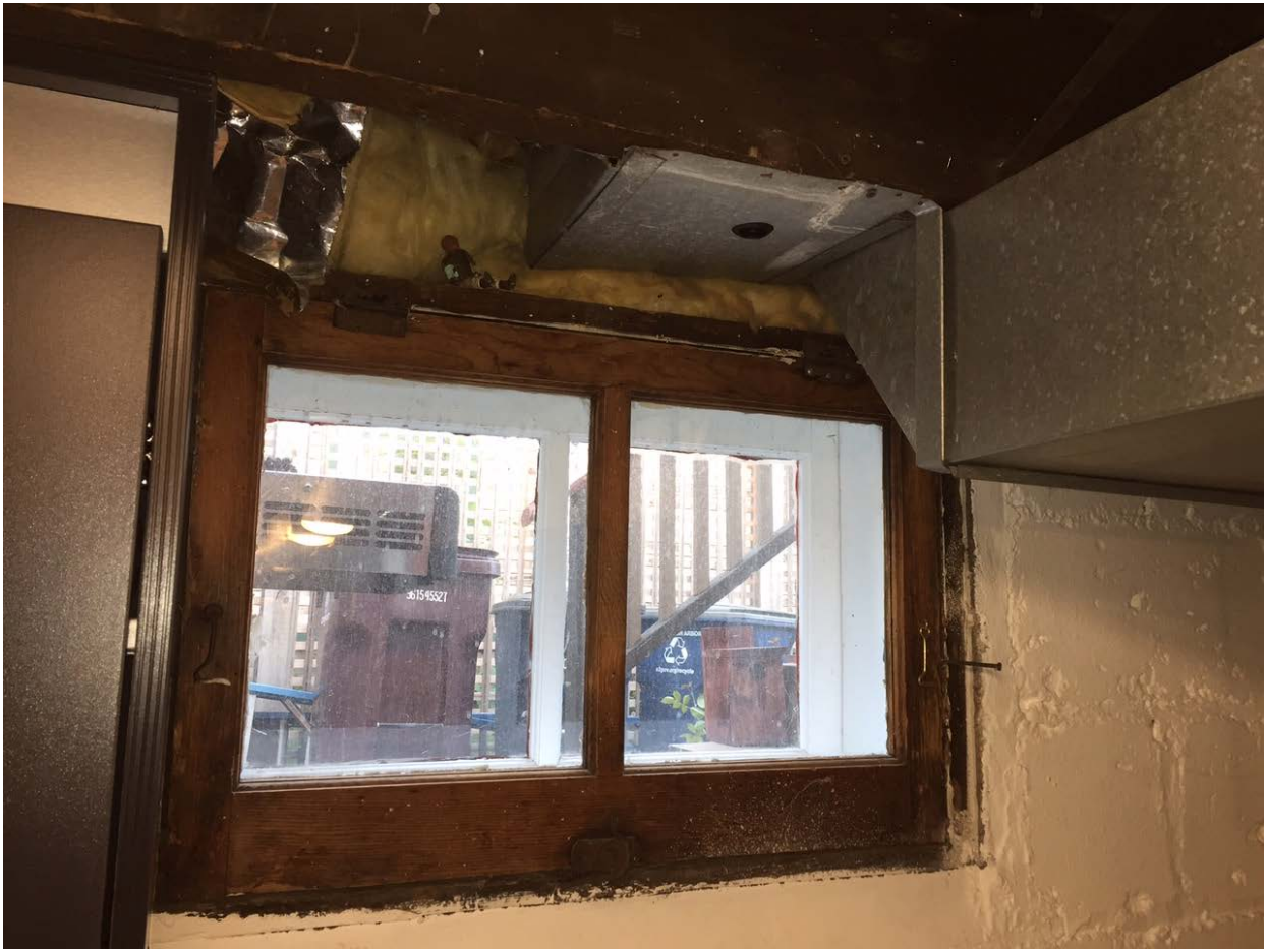
Image #3 - West basement window exterior view
