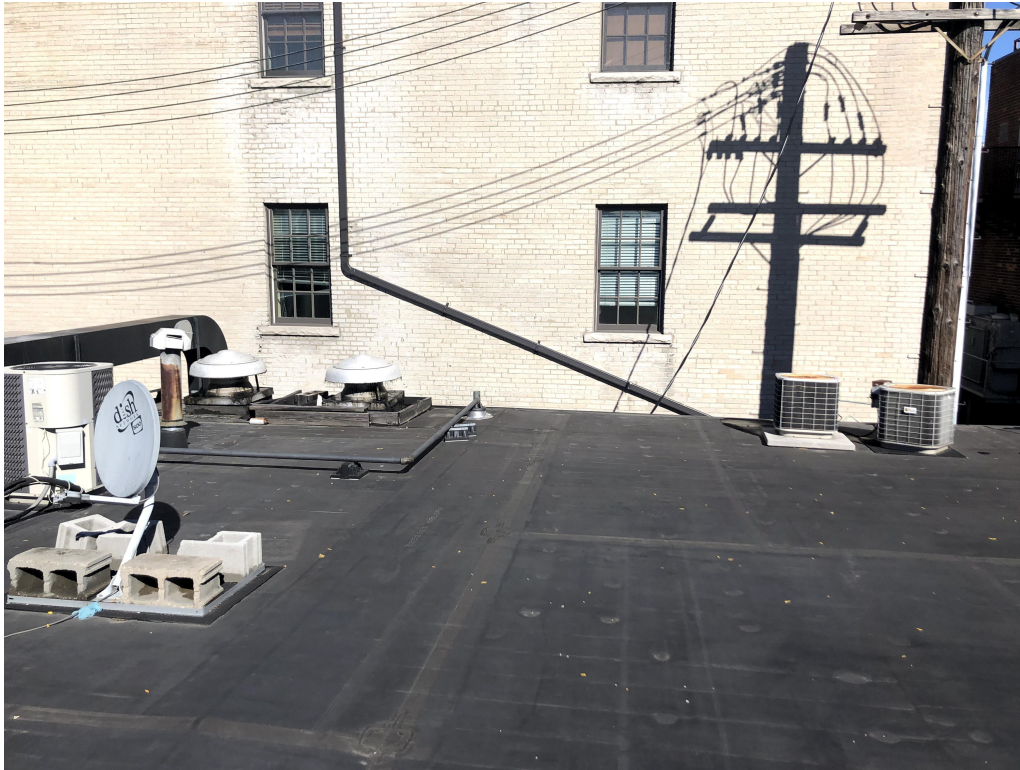
Photo 11: North Roof View
