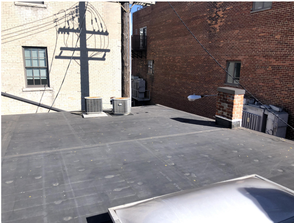
Photo 12: Northeast Roof View
