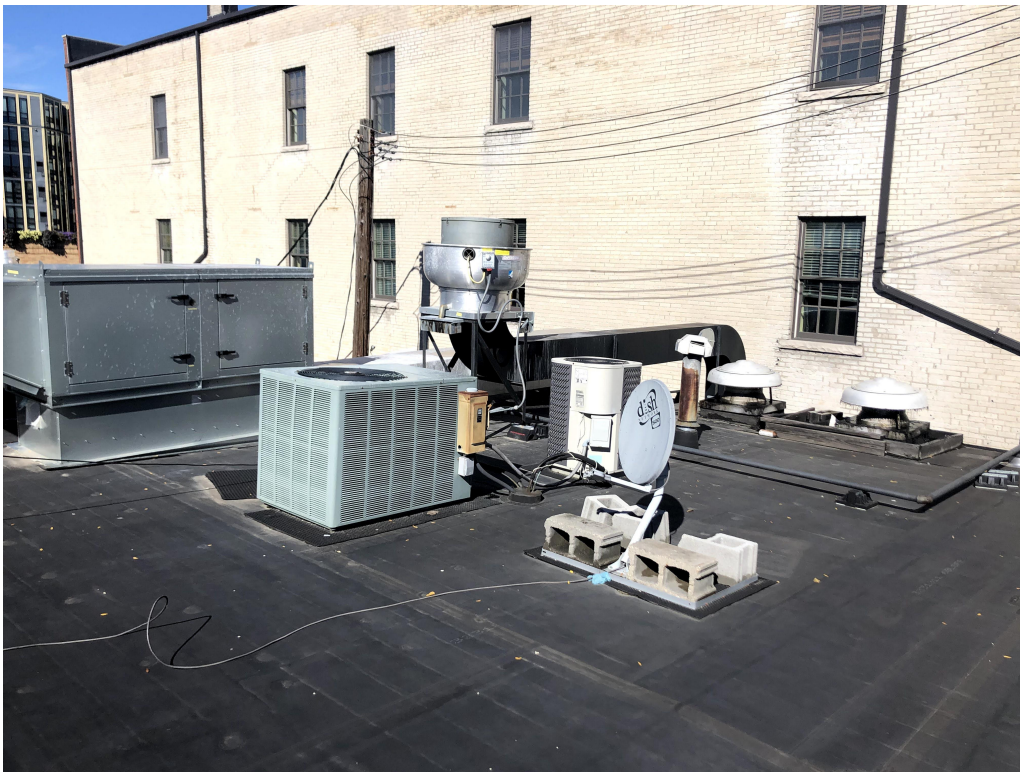
Photo 10: Northwest Roof View
