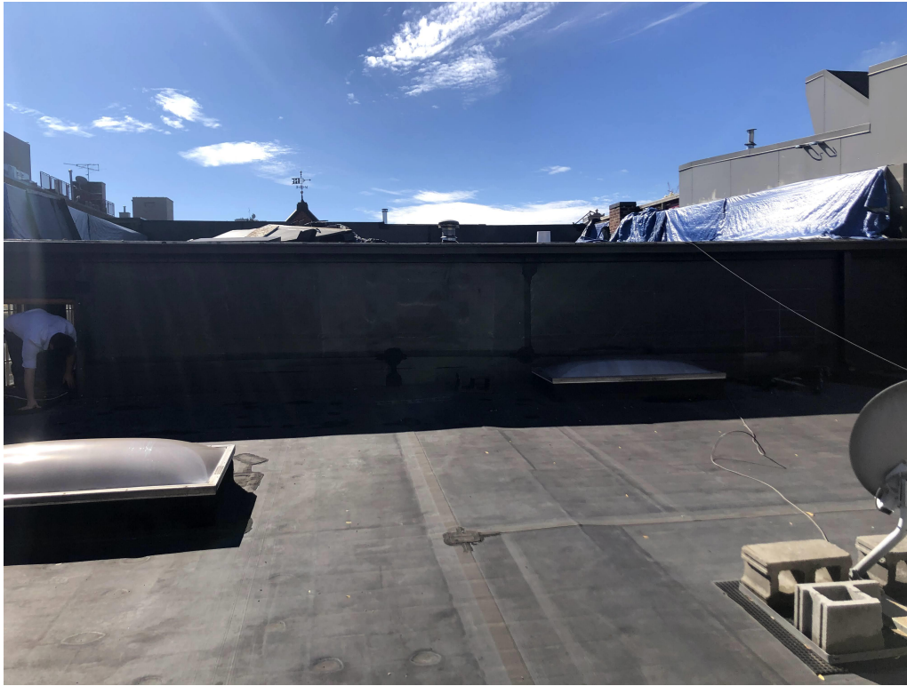
Photo 9: South Roof View
