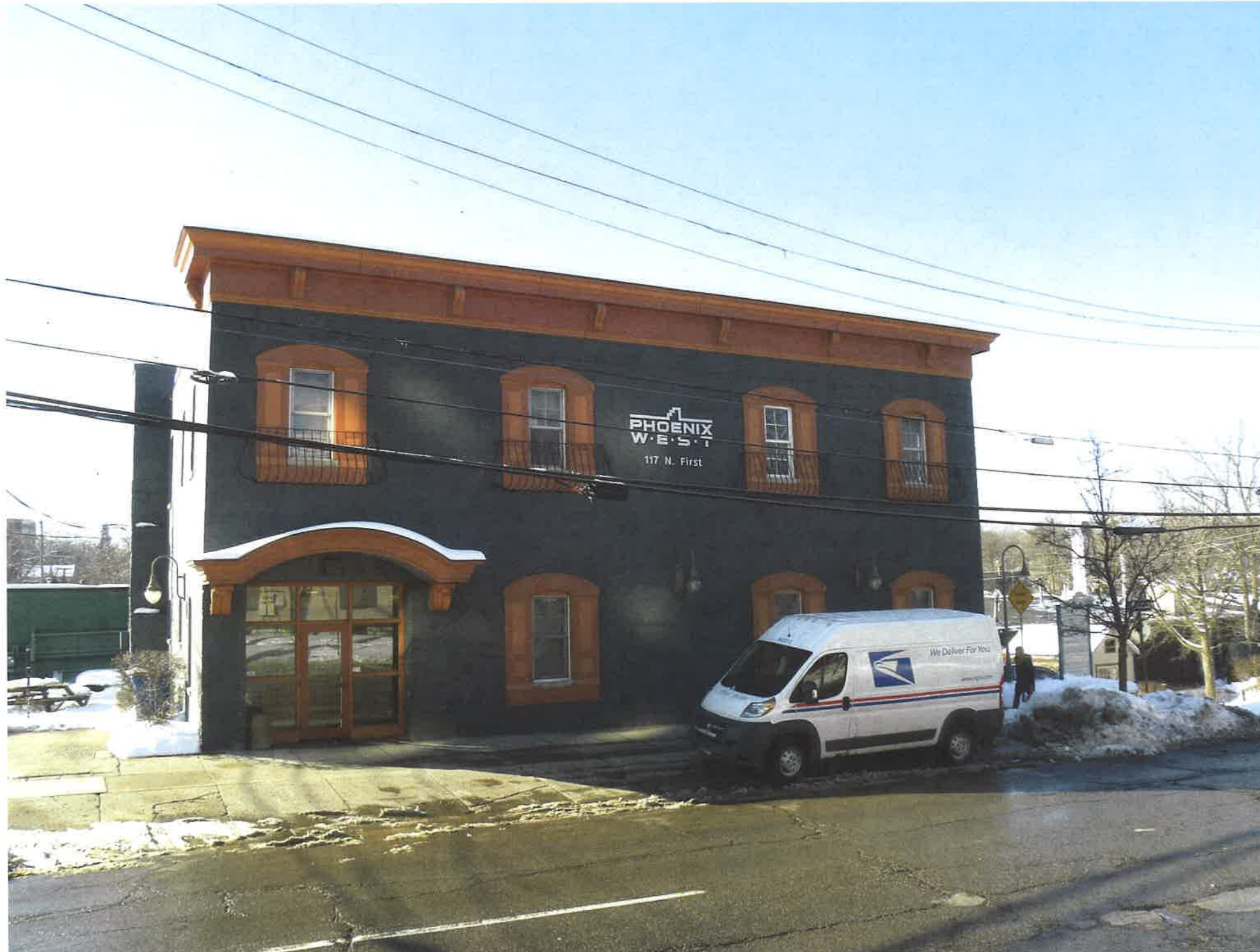
Phoenix W.E.S.T. located on the Southwest corner of North First Street and West Ann Street
