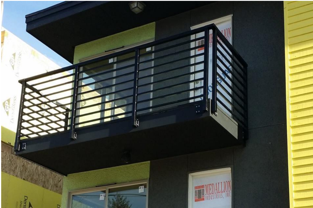
Metal balcony handrail example in anodized aluminum or powder coated steel
