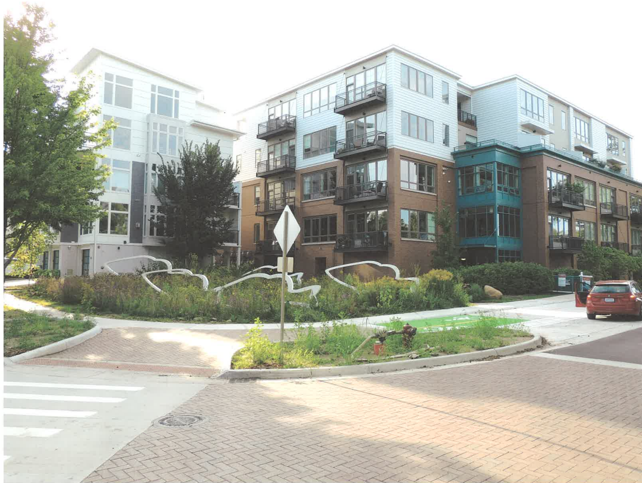
KINGSLEY PARKSIDE CONDOMINIUMS
