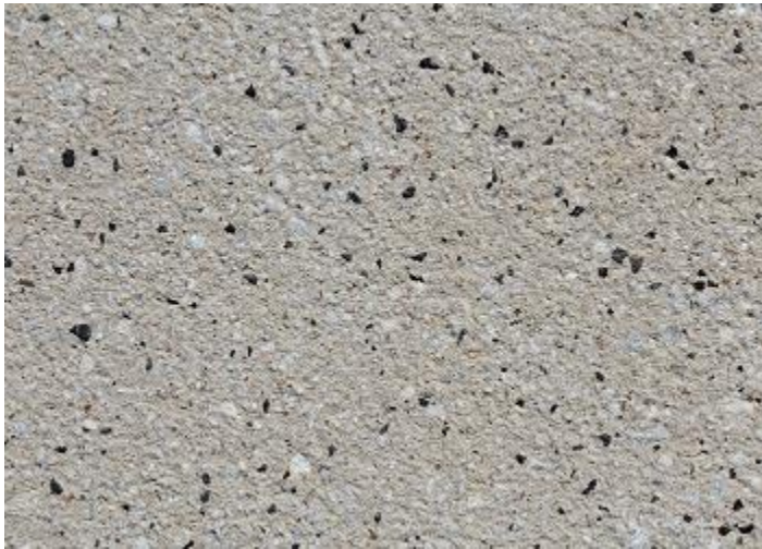
Sandblasted concrete landscape planter and foundation wall finish
