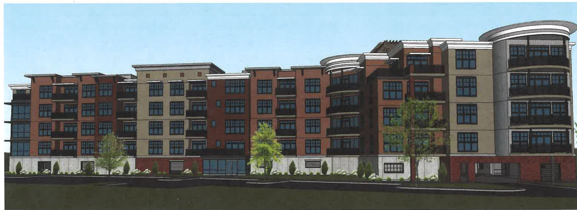
Kingsley Condos located on the north corner of North 1st Street and West Kingsley Street (under construction)
