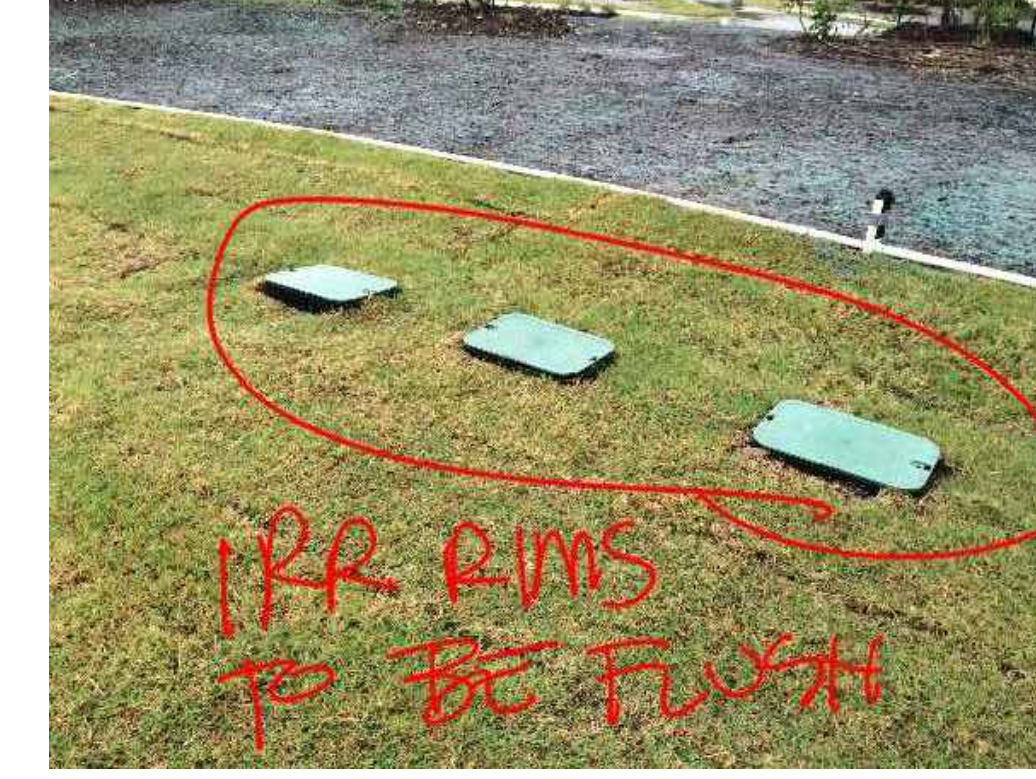
NOT STANDARD - IRRIGATION VALVE LIDS TO BE FLUSH WITH ADJACENT LAWN AREAS
