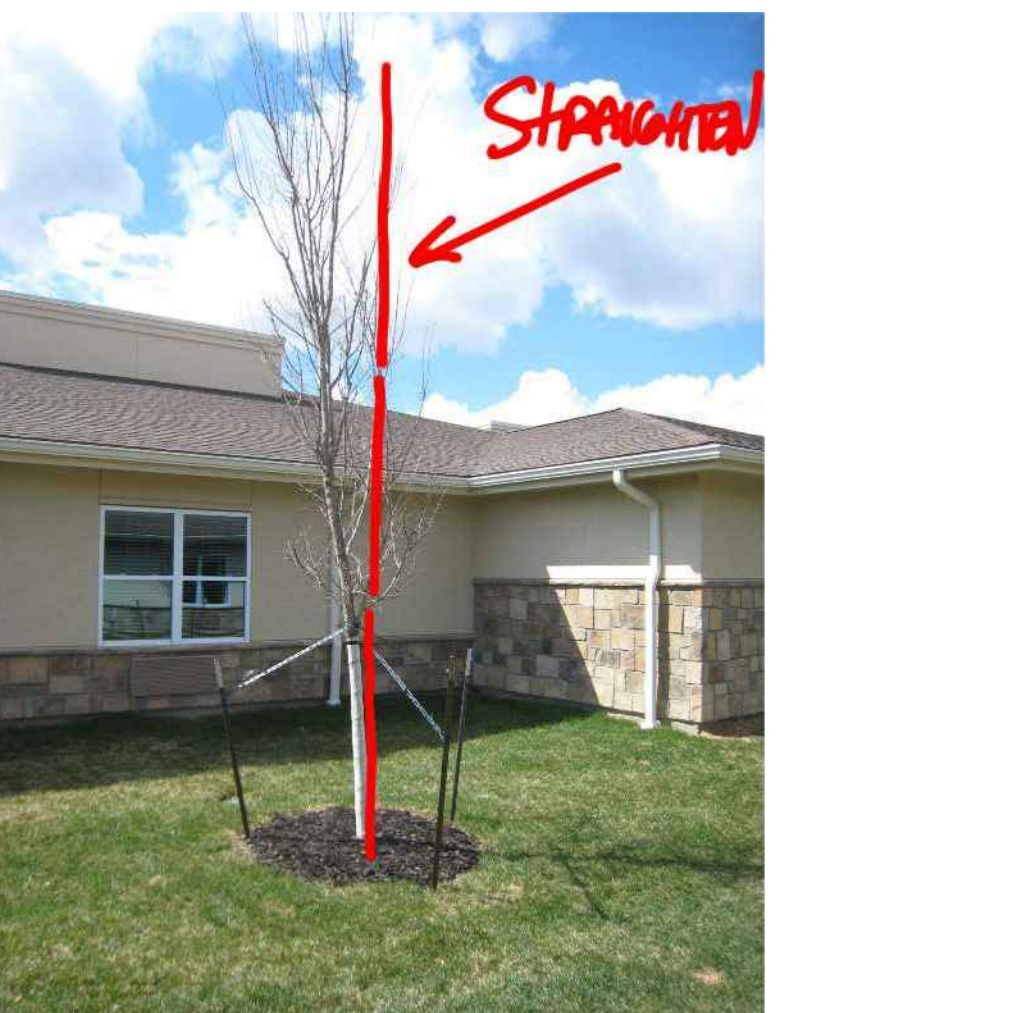
NOT STANDARD - CROOKED PLANTS. INSTALL TREES AND SHRUBS PLUMB, AND DO NOT BURY TRUNKS WITH EXCESSIVE MULCH
