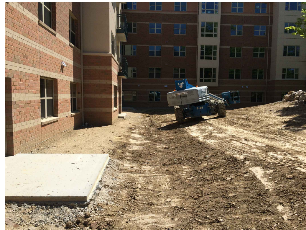
PRIOR TO TOPSOIL BEING INSTALLED IN LAWN AREAS
