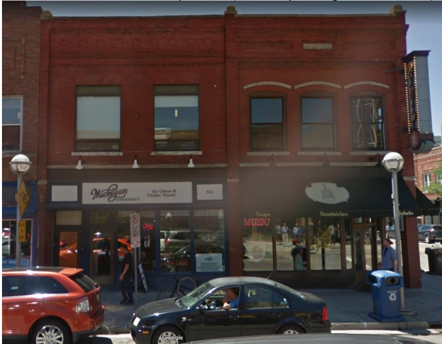
Front of 300 S. State, July 2018 (courtesy Google Streetview)
