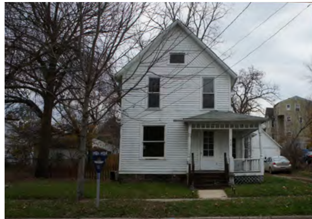
412 North First Street (to be demolished)
