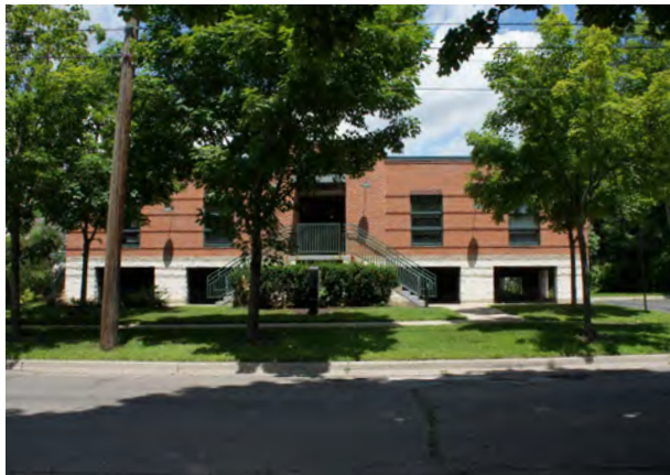
214 Kingsley Street offices raised above flood elevation
