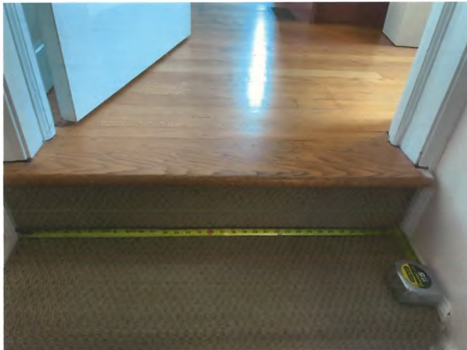
Picture 4: Width of staircase is 33.5"
