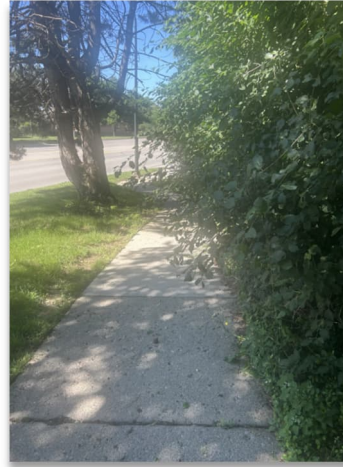
Overgrown Vegetation along Sidewalk
