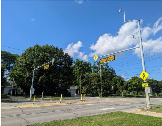
Figure 23 – Pedestrian Hybrid Beacon Crossing Along Plymouth Road West of Green Road
