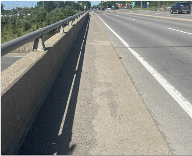
Gravel Along US-23 Overpass
