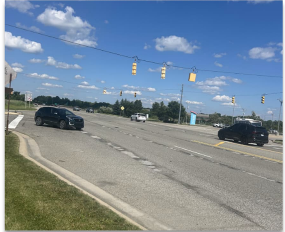
Plymouth Road and Southbound US-23 Intersection
