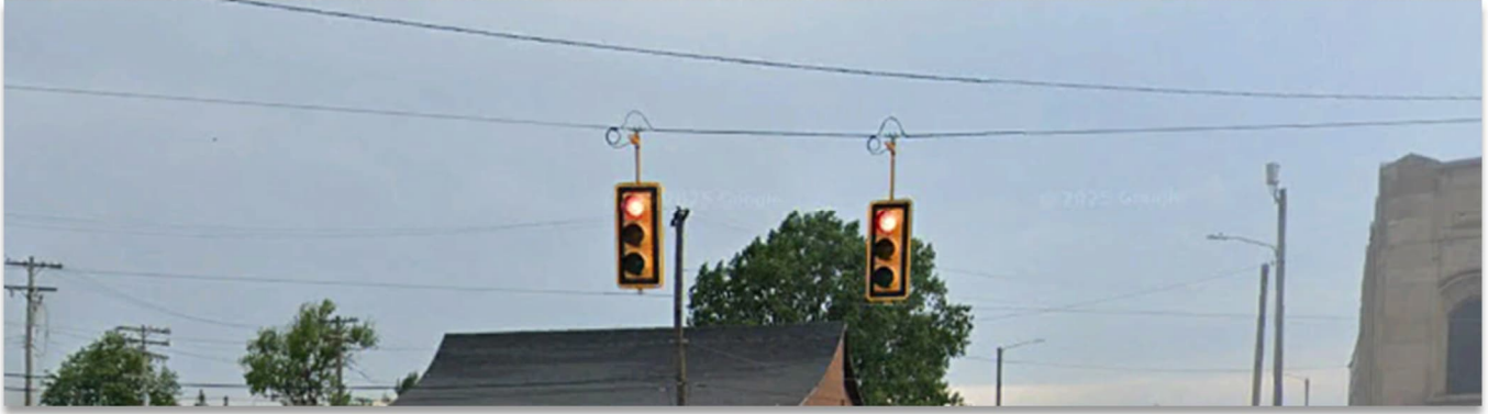
Figure 33 – Example of Backplates and Tethers – Detroit, Gratiot Avenue & Chene Street (Source: Google Earth Streetview)
