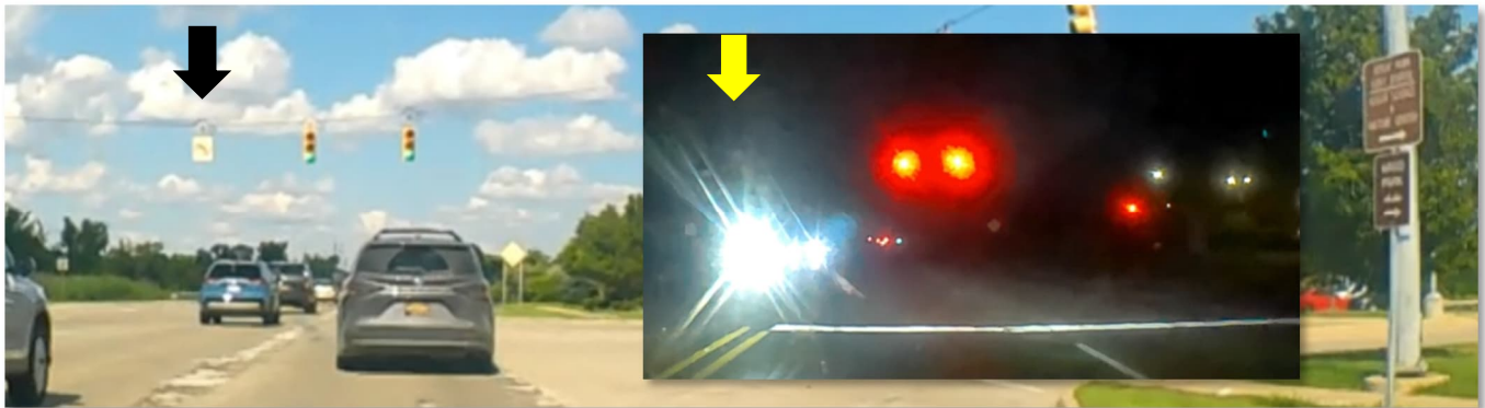
Figure 31 – Non-illuminated Left Turn Case Sign at Southbound US-23 On-Off Ramp Intersection
