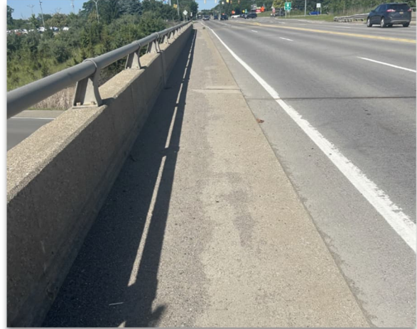
Sidewalk along Bridge over US-23
