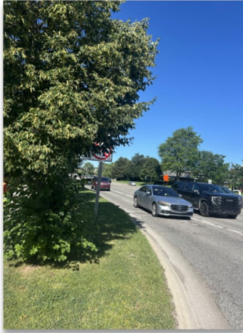
Vegetation Obstructing Visibility at Southbound US-23 On Ramp
