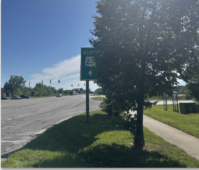
Vegetation Obstructing Signage
