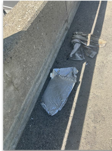
Debris Along US-23 Overpass
