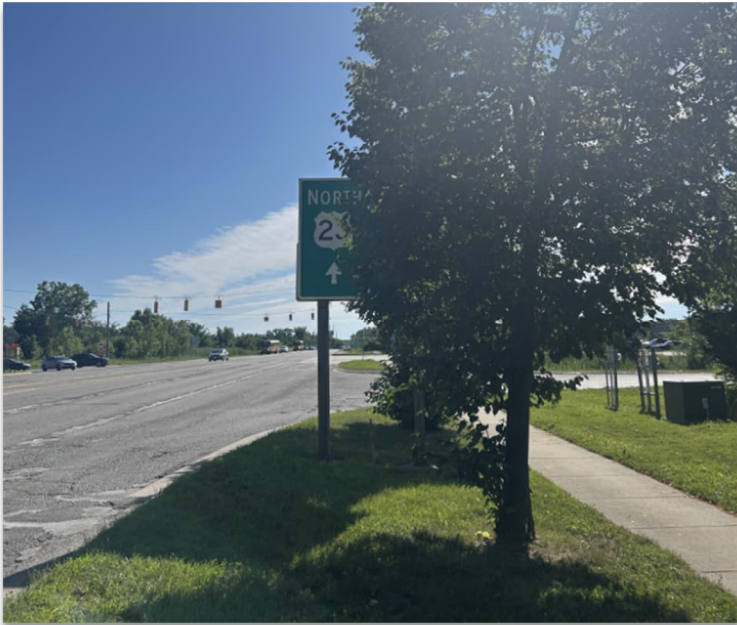
Vegetation Obstructing Signage
