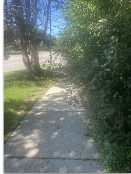
Vegetation Obstructing Sidewalk
