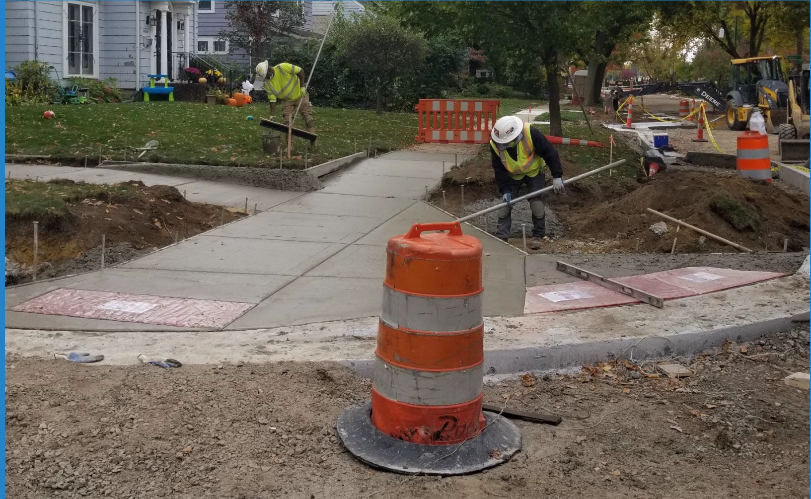
ADA Sidewalk Installation on Granger Ave.
