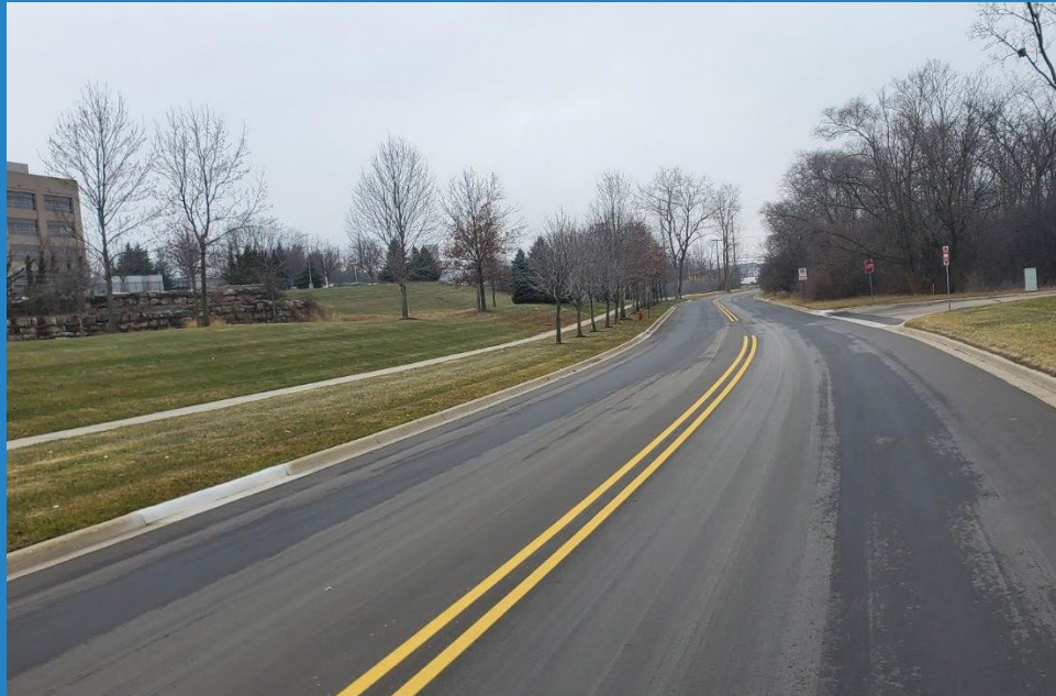
Street Resurfacing on Boardwalk Drive
