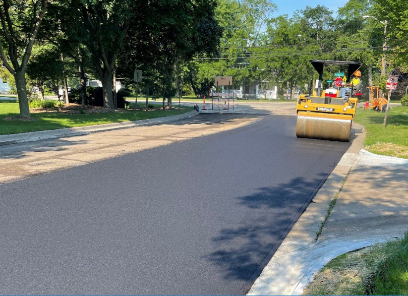
Local Street Paving on Crestland Drive
