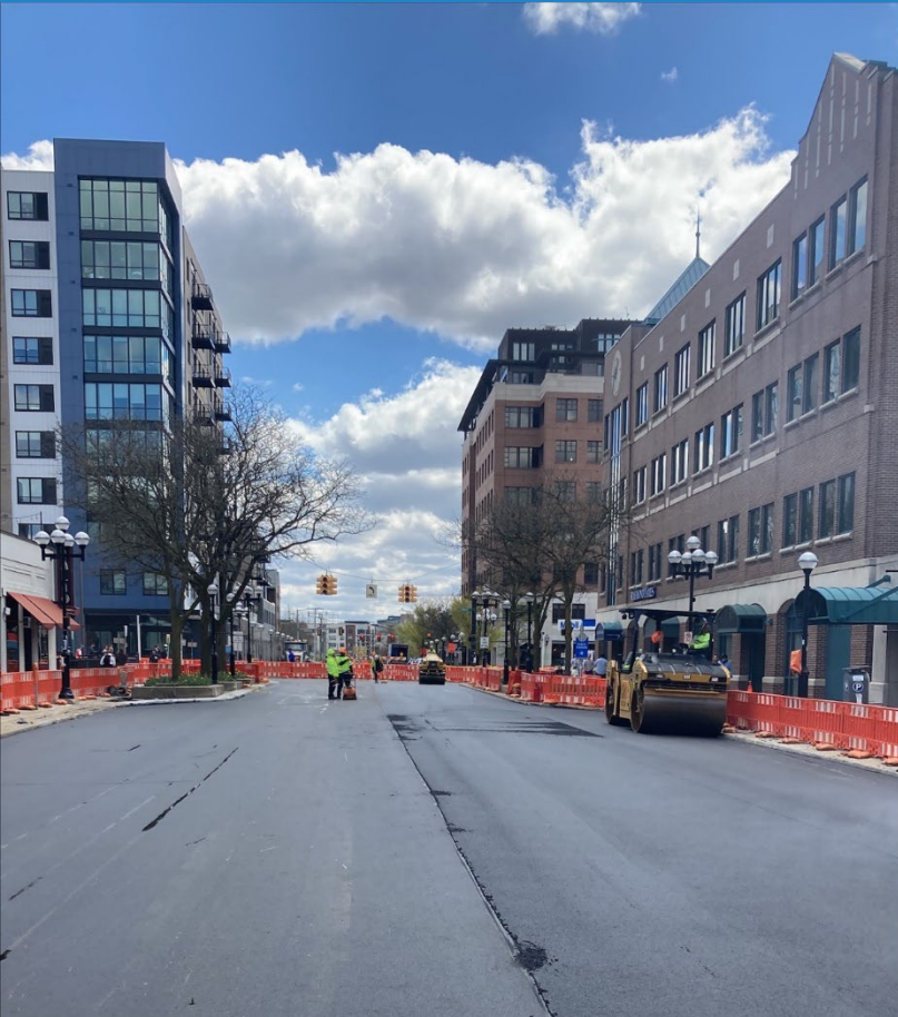
Main Street Paving, 2023
