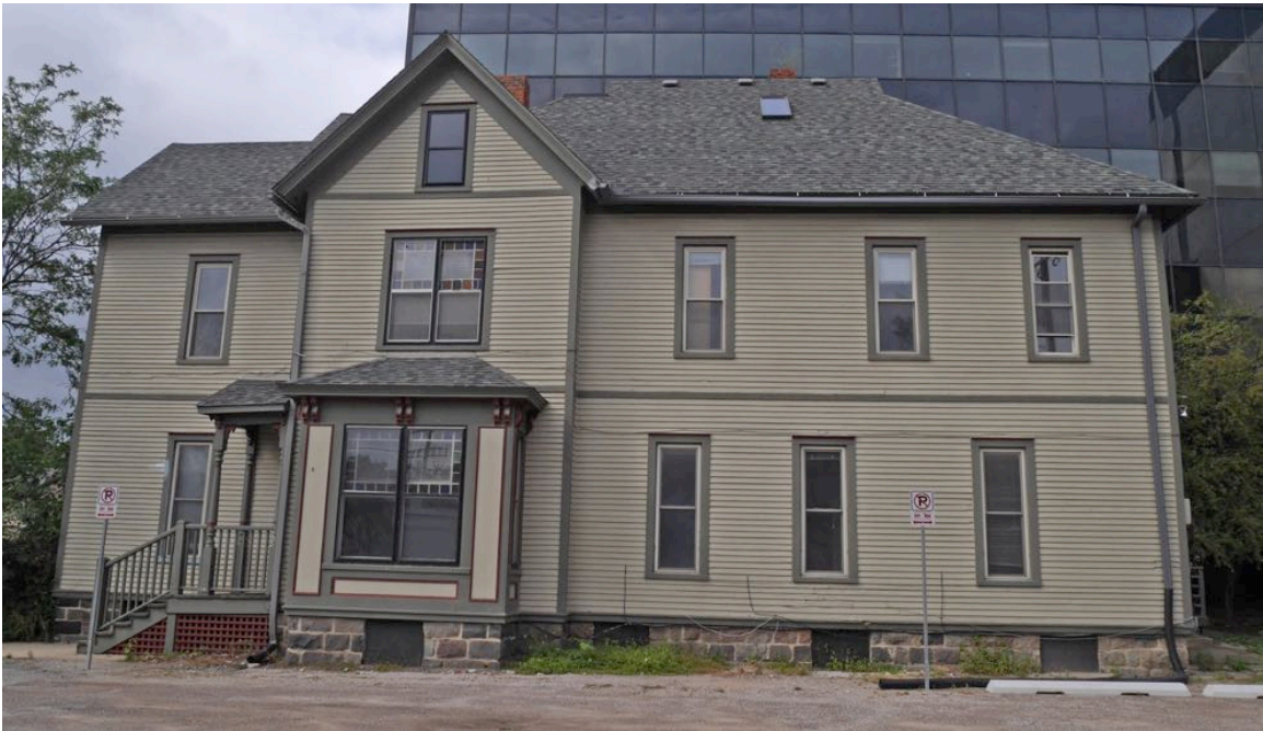
Photo No. 17 (image No. 46): South elevation faces a vacant lot. Bay window and porch are in very good condition. From this view it is also easy to see that the asphalt roof shingles are new.
