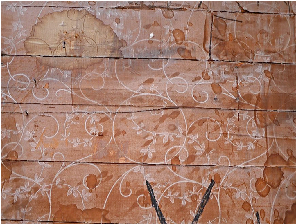
Photo No. 10 (image No. 29): Detail of wallpaper that covered the boarded sloped ceiling in the front/west room of the attic.
