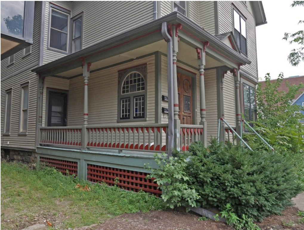
Photo No. 14 (image No. 38): View of front porch showing intact unique railing system, Italianate brackets, and lattice.
