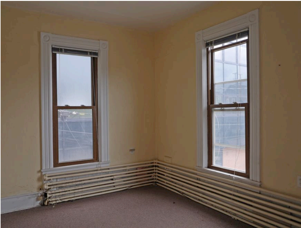
Photo No. 7 (image No. 21): Southeast corner windows of back bedroom (BR #6 on second floor sketch plan) with unusual radiant heating pipes below them.
