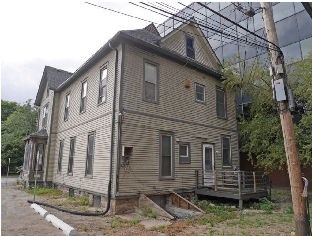
Photo No. 16 (image No. 44): East elevation is where most change has occurred. The original "back" door has been changed to a small window, and a new door added that leads into the modern kitchen. Cellar door cover is missing.
