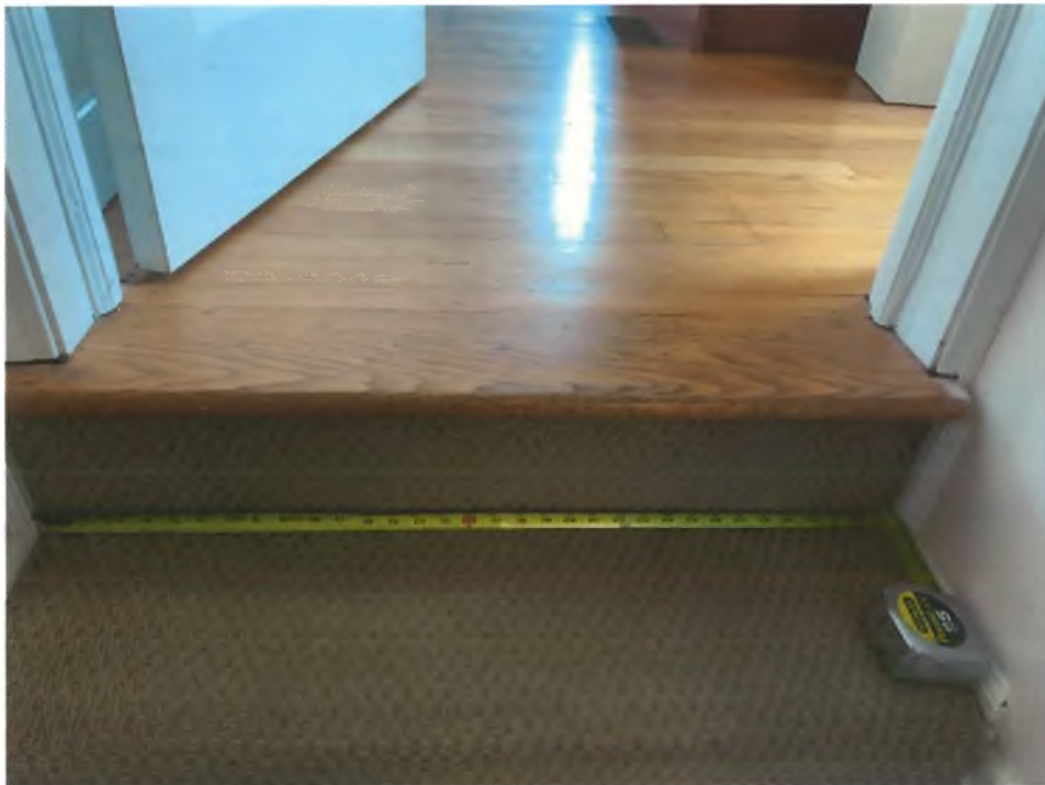
Picture 4: Width of staircase is 33.5"
