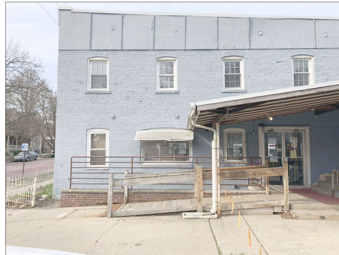
VIEW OF A PORTION OF THE EXISTING NORTH ELEVATION
