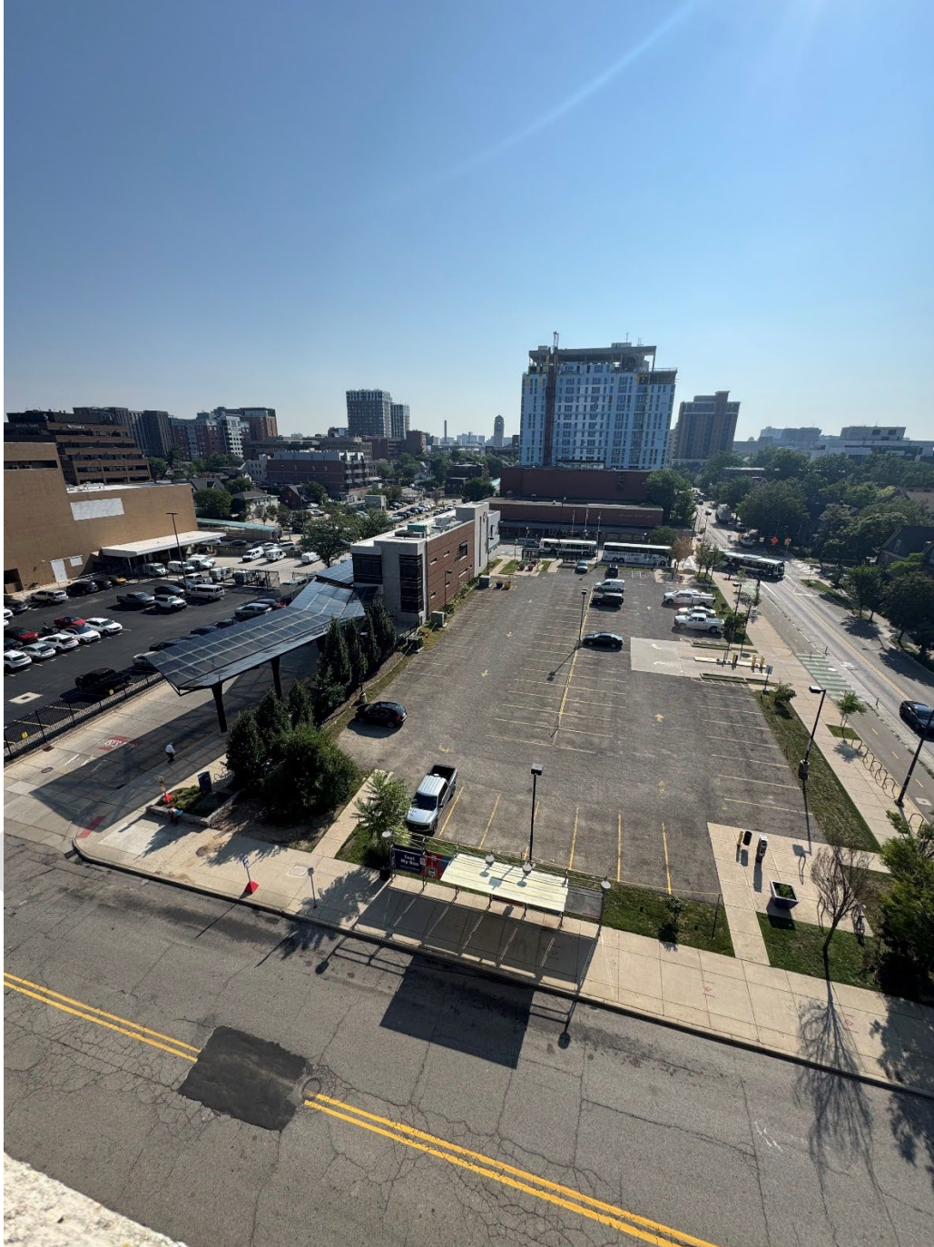
East-facing View of 350 S Fifth Ave
