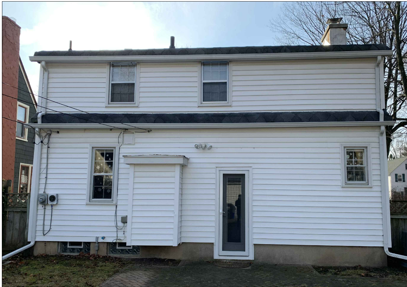
1. REAR VIEW OF EXTERIOR OF EXISTING HOUSE
