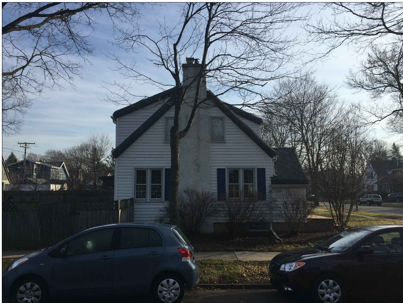
2. SIDE VIEW OF THE EXISTING HOUSE
