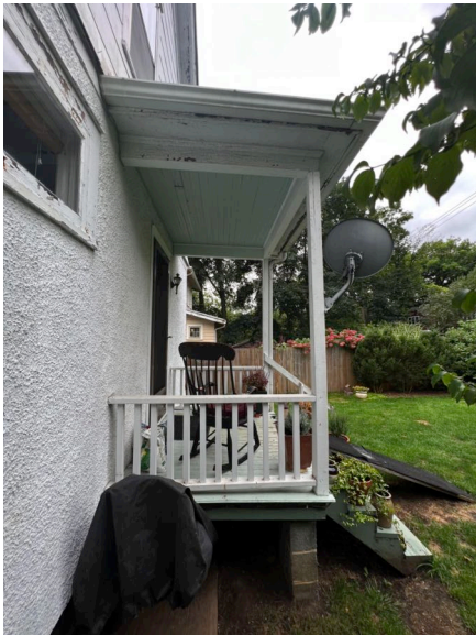
Side Elevation of the existing rear porch
