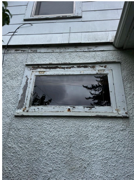
Close up of the awning window to be removed
