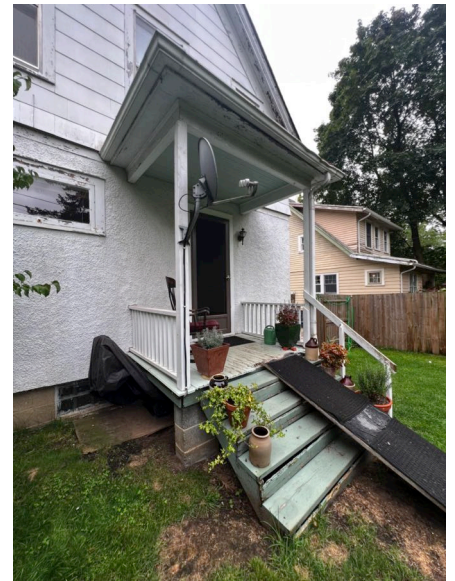
Corner view of the existing rear porch
