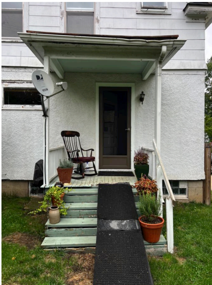
Western Facing Existing Rear Porch
