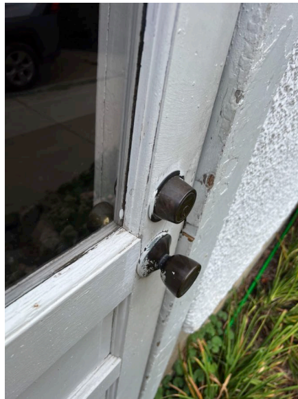
Existing door glazing is made of plexiglass; Existing hardware is modern
