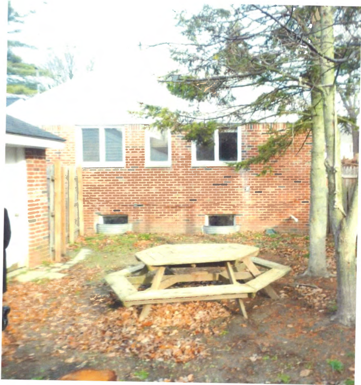
Almost no grass, holes in the ground, debris, no AC
