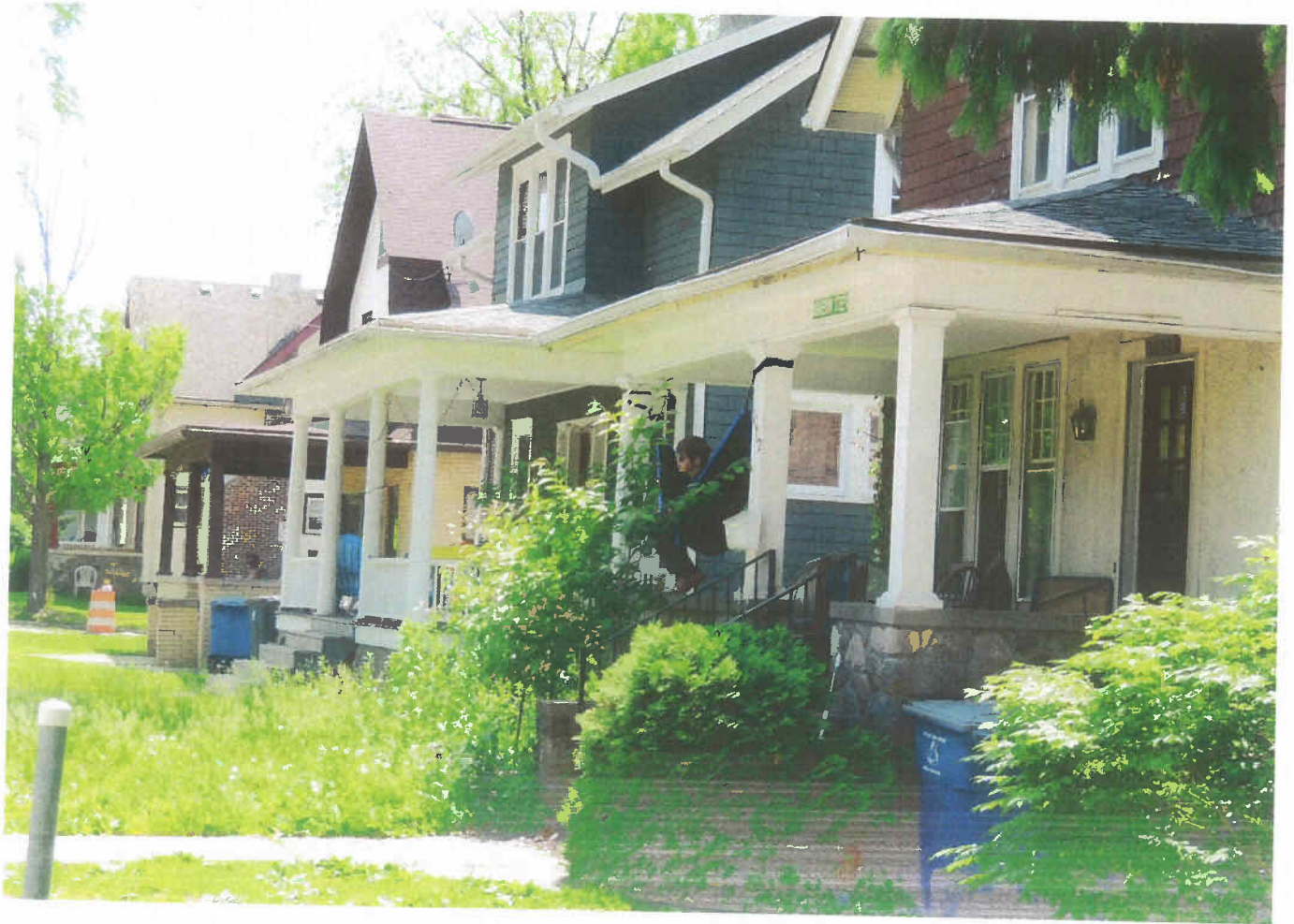
TYPICAL PORCH ENCROACHMENTS INTO FRONT SETBACKS ALONG PACKARD IN NEIGHBORHOOD OF 918 PACKARD
