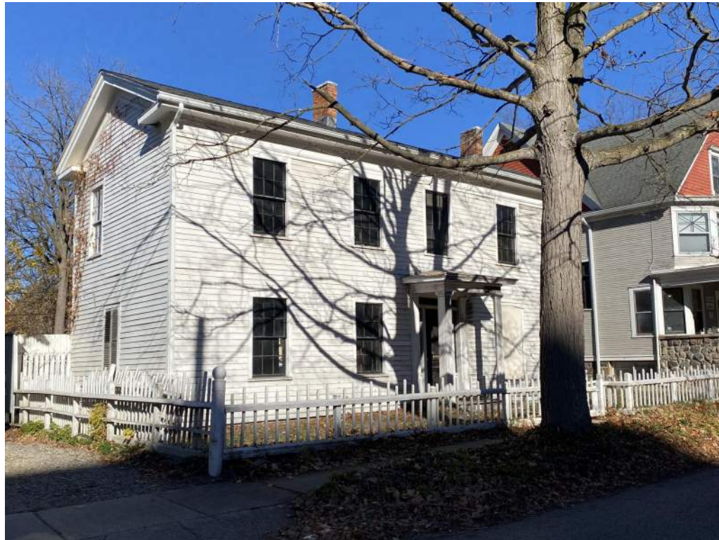
View of Front (South)
