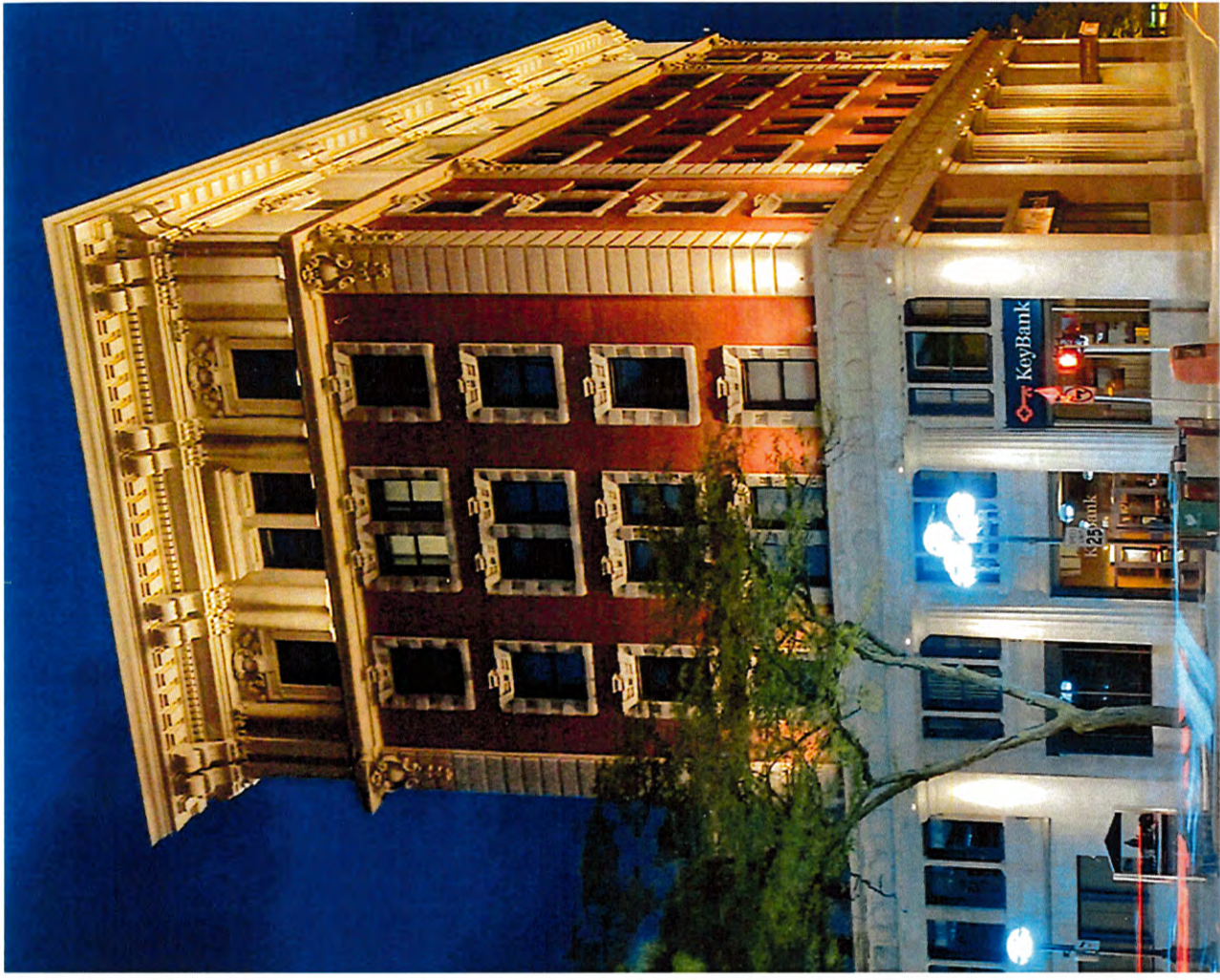
KeyBank Building - After
