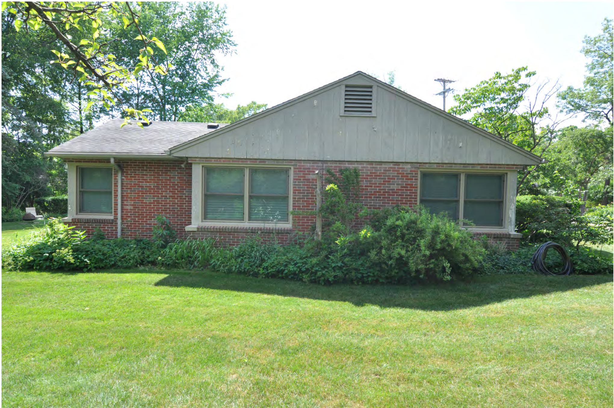
EAST ELEVATION OF 1001 VESPER STANDING IN FRONT YARD SETBACK FROM MINGLEWOOD WAY
