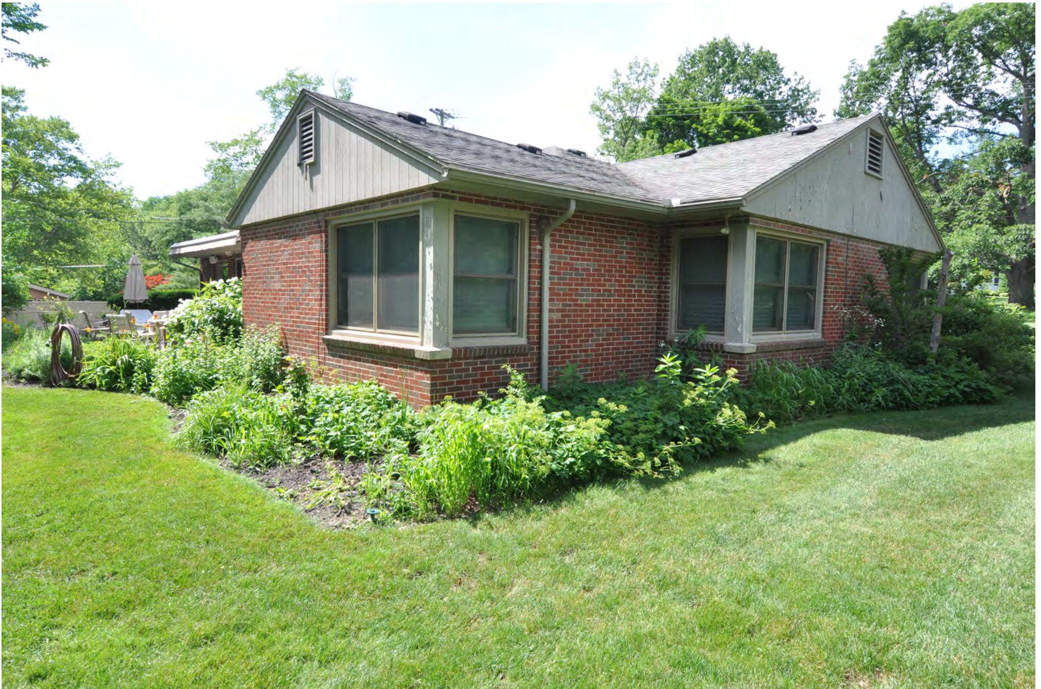
SOUTH / EAST ELEVATION OF 1001 VESPER STANDING IN FRONT YARD SETBACK FROM MINGLEWOOD WAY
