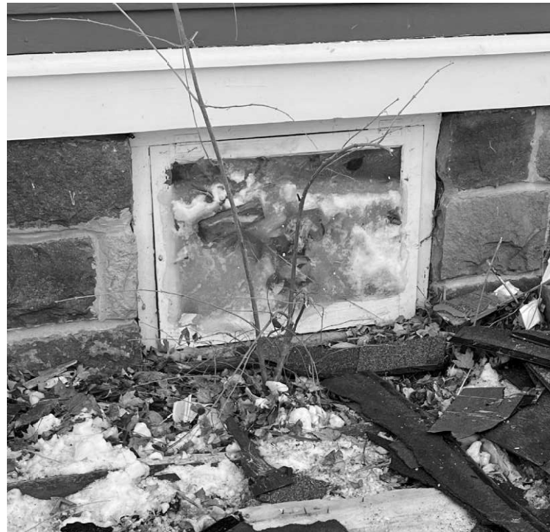
BASEMENT WINDOW - EAST SIDE TOWARD FRONT PROPOSED TO BE REPLACED AS EGRESS WINDOW EXISTING WINDOW IS WOOD (2'-6" WIDE BY 2'-0" HIGH) EXISTING WINDOW IS A HOPPER WITH AN AWNING STYLE STROM WINDOW. IT APPEARS TO BE ORIGINAL.
