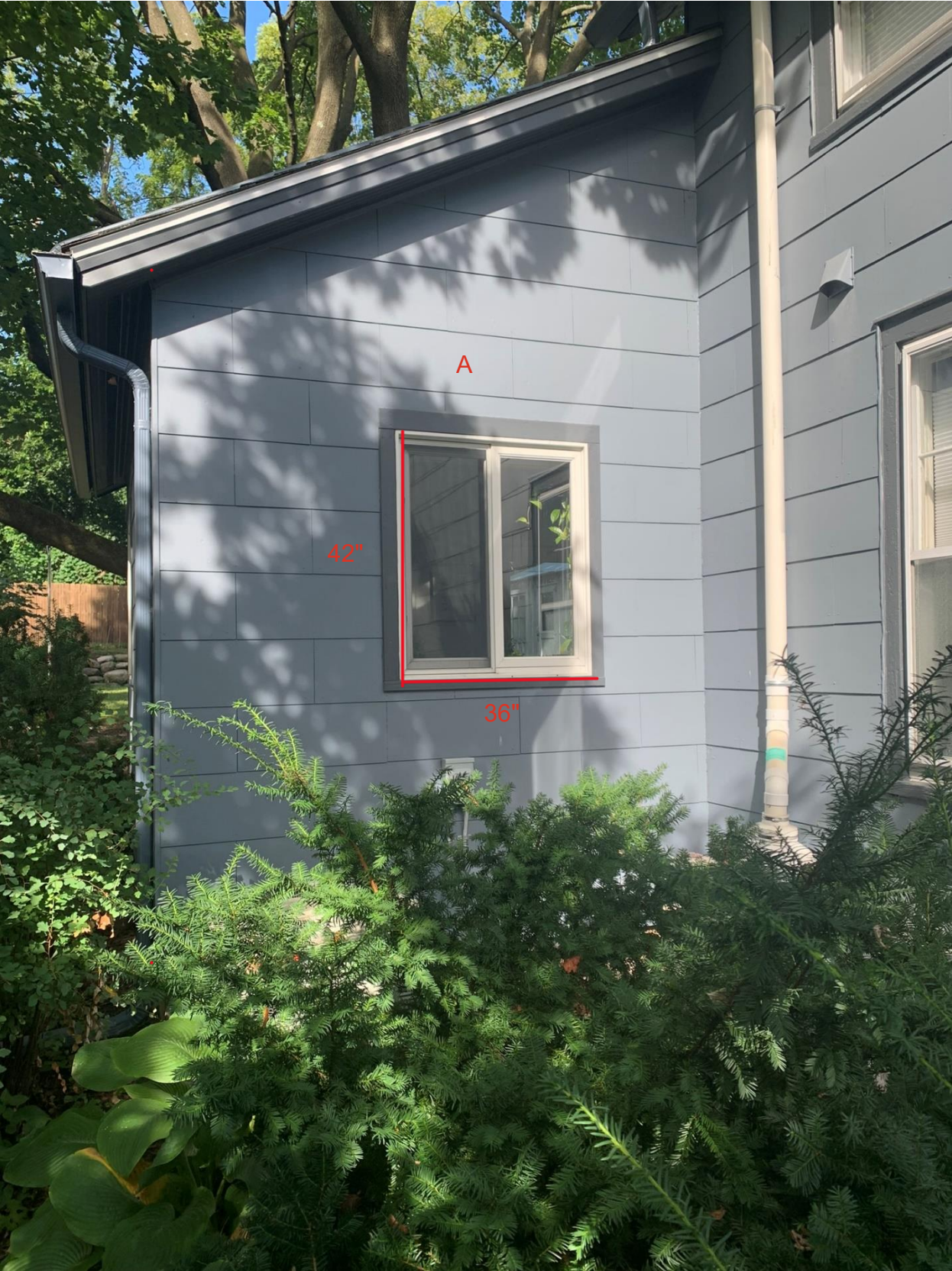
Kitchen east. Trim is 3.5" on top, 2.5" on sides, 1.5" on bottom.
