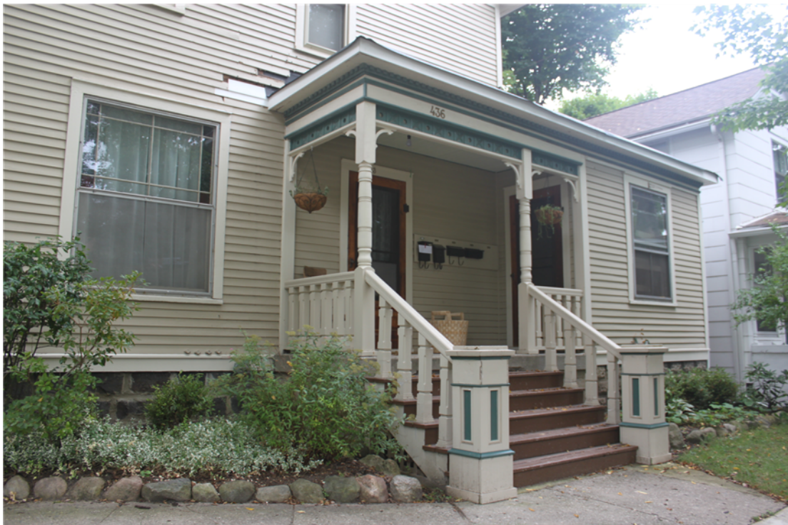
Detail of Main house front porch
