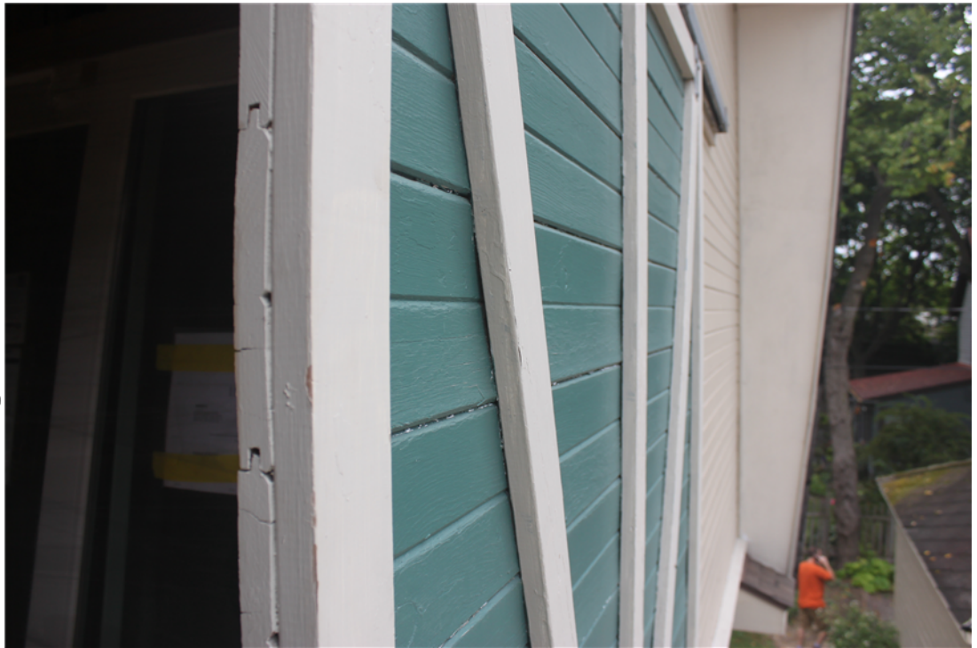
Existing T&G siding (Pattern #116 ) on Duplex
