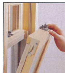
Sash tilting freely into the room
