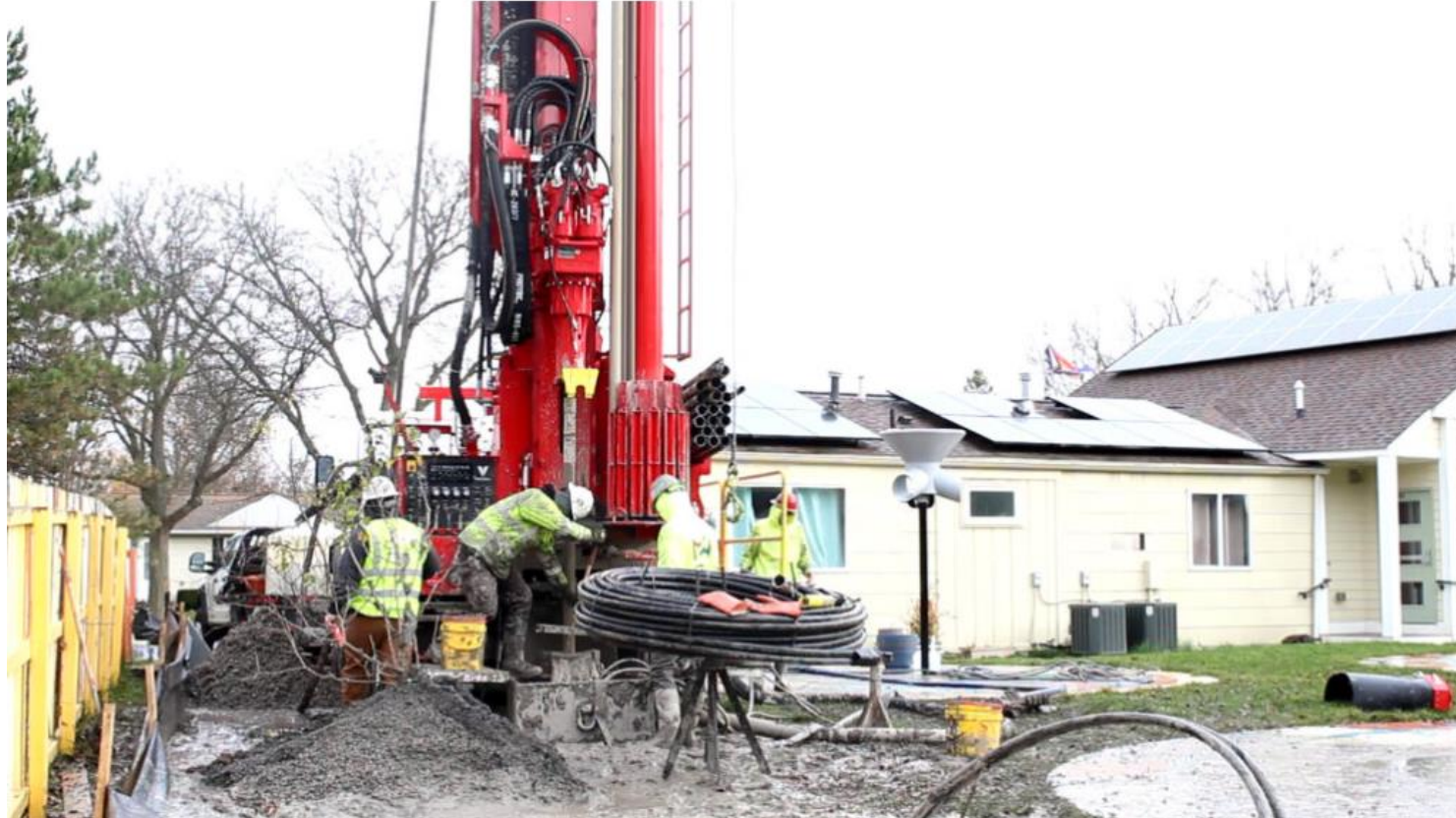
Geothermal system installation at Bryant Community Center
