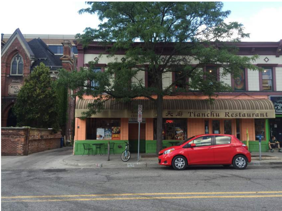
Existing Facade Conditions
