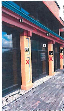
2 Exhibit C - Southeast Deck View EX-C2
