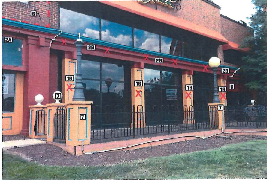
3 Exhibit C - Southeast Exterior View EX-C2
