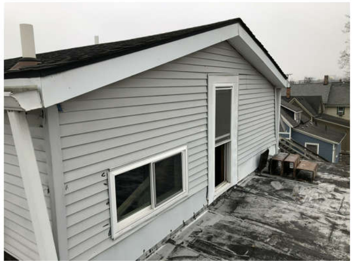
(E) WEST VIEW OF ROOF
