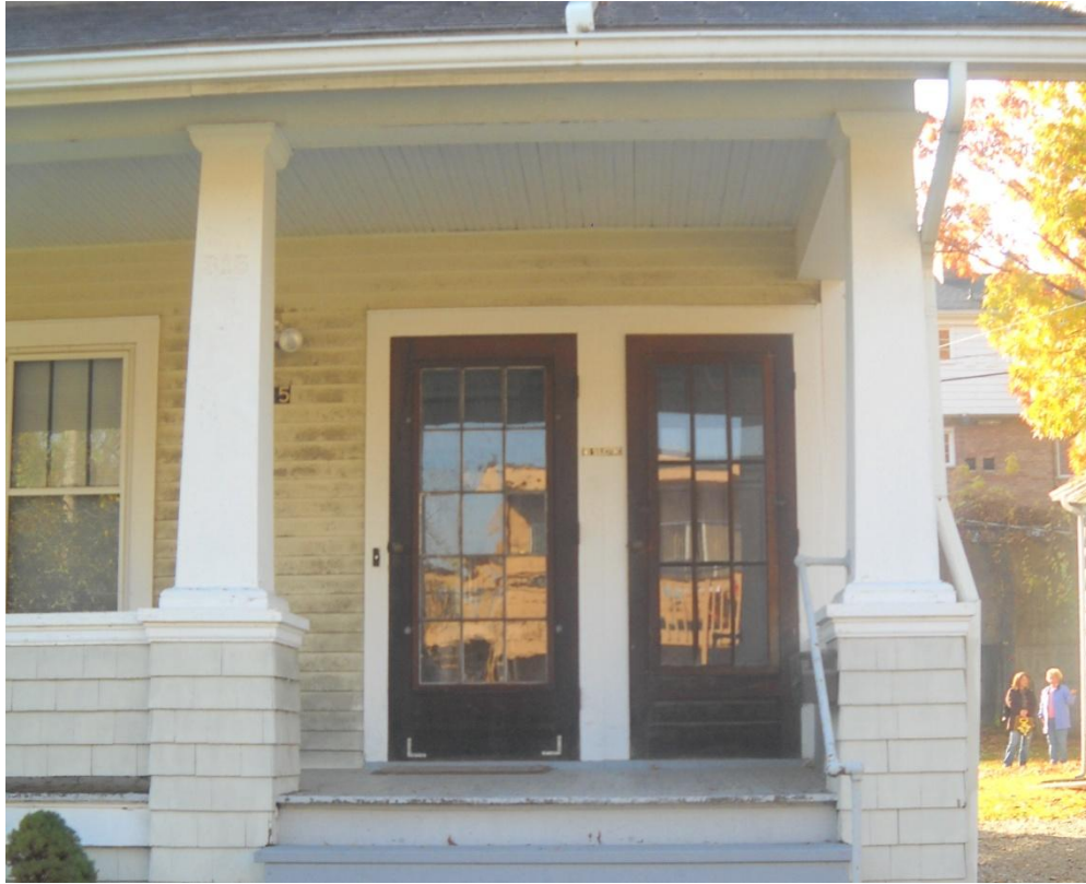
Existing Front Doors
