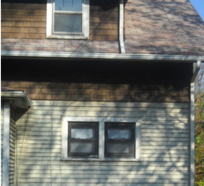
Existing aluminum replacement windows with aluminum storm windows
