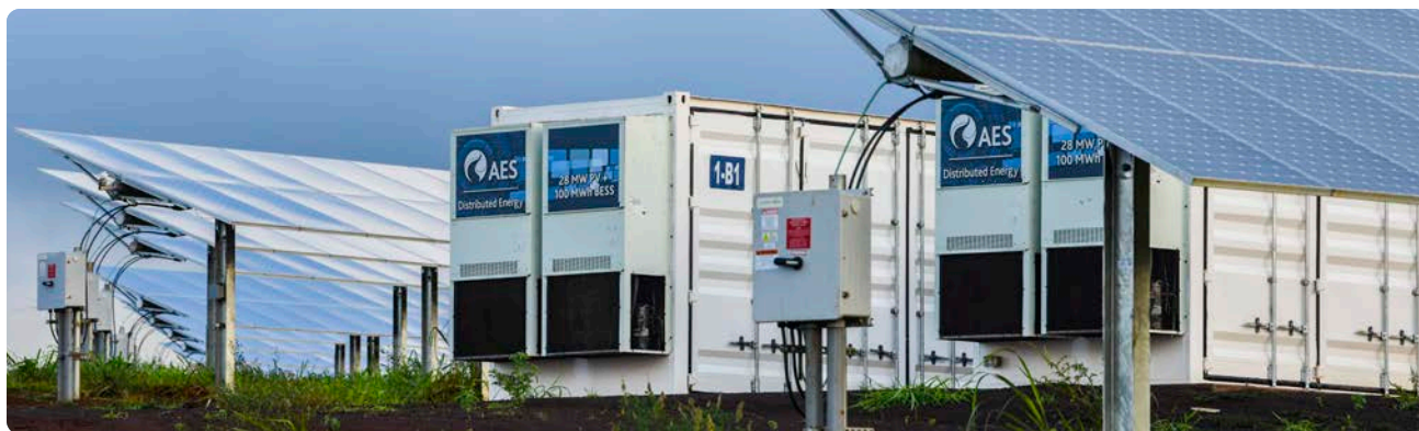
The AES Lawai Solar Project pairs BESS with solar photovoltaic energy to increase grid reliability and energy independence on Kaua’i Island, HI (Photo: Dennis Schroeder / NREL 57997)
