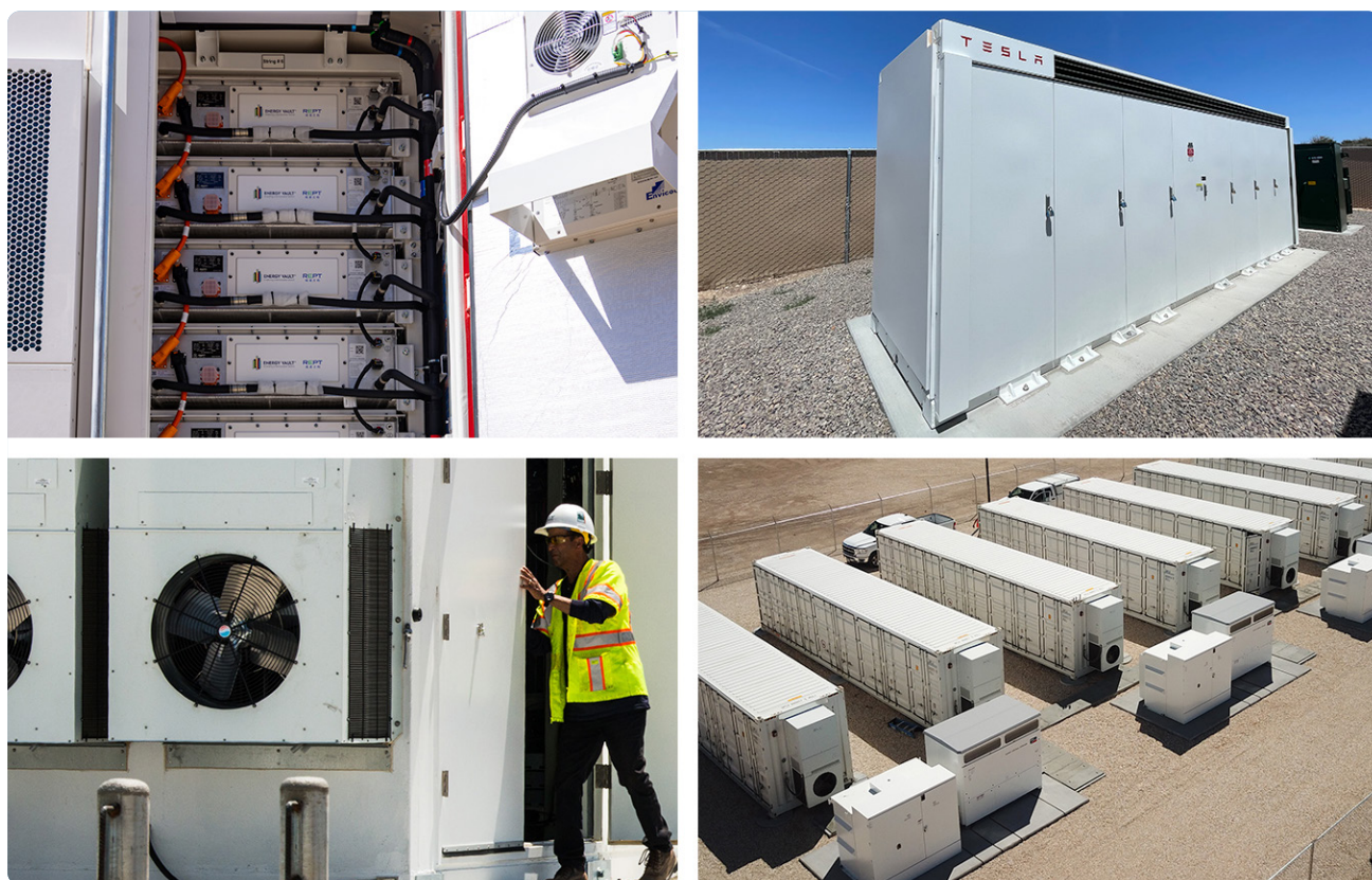
(Clockwise from top left) Battery modules (Photo: Agata Bogucka / NREL 88687); Battery enclosure (Photo: Laura Beshilas / NREL 88842); Enclosures, inverters, and transformers (Photo: Key Capture Energy); Thermal management system (Photo: Dennis Schroeder / NREL 50688)
