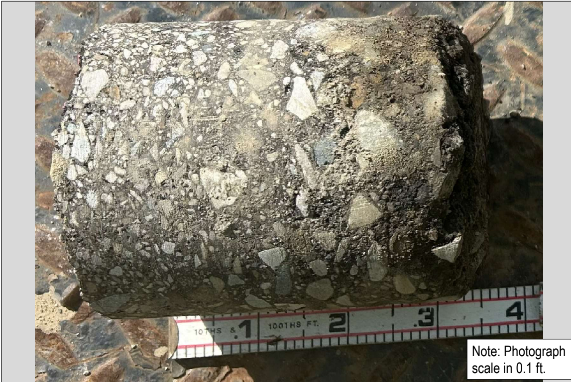
Photo 14: SB-2026-121 (Packard St.): 4-inch Asphalt
