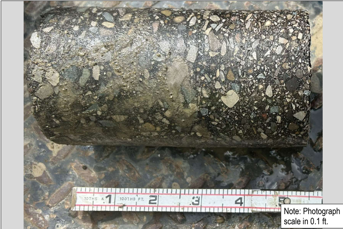
Photo 12: SB-2026-119 (Packard St.): 6.5-inch Asphalt
