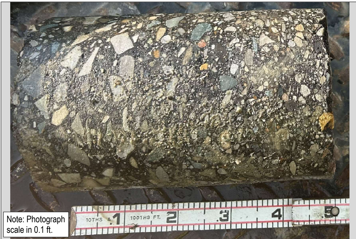
Photo 15: SB-2026-122 (Packard St.): 6-inch Asphalt
