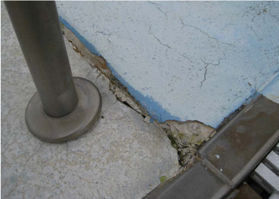
Spalling concrete
