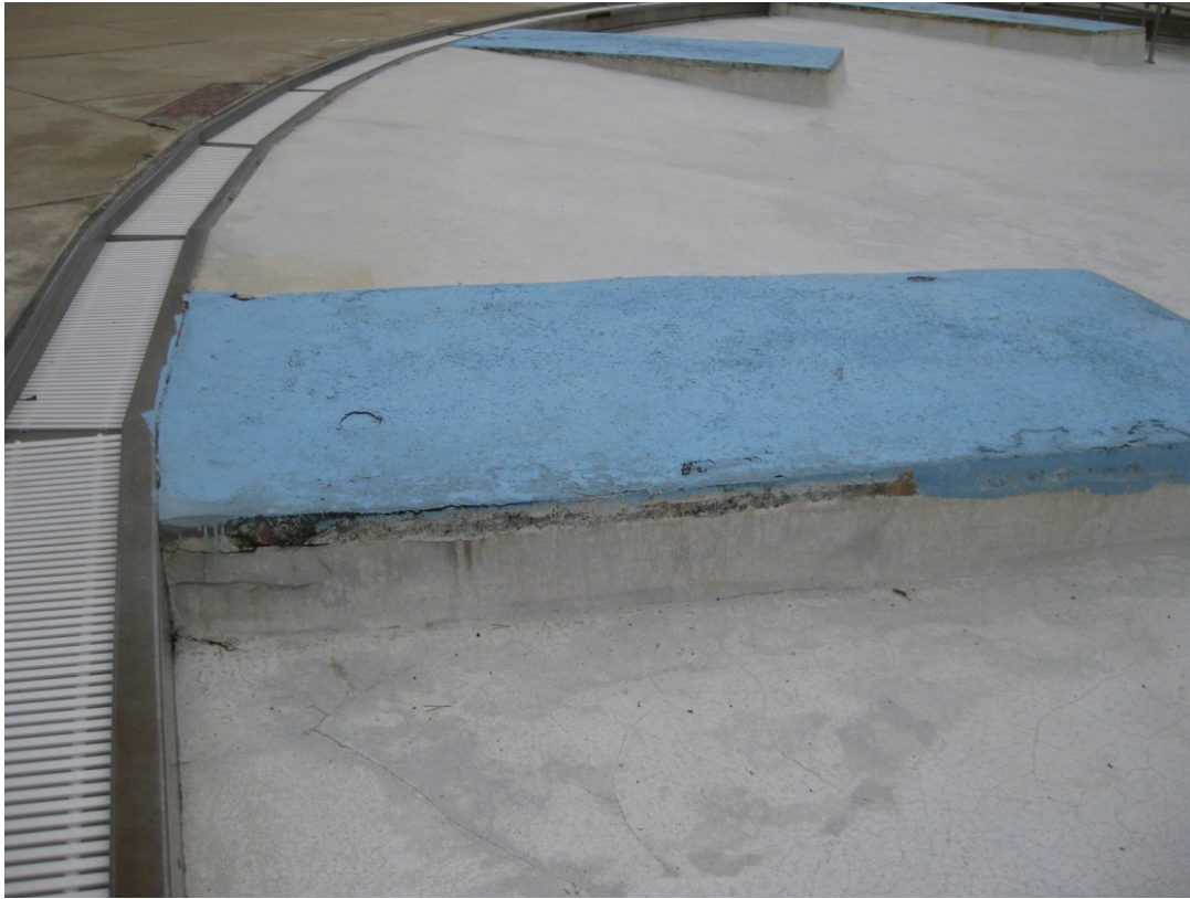
Concrete pads in wading pool
