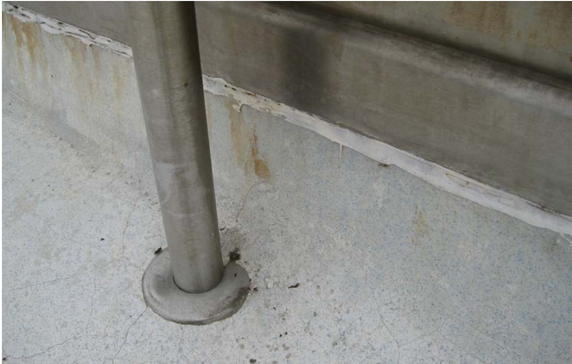
Install base cones on handrail system
