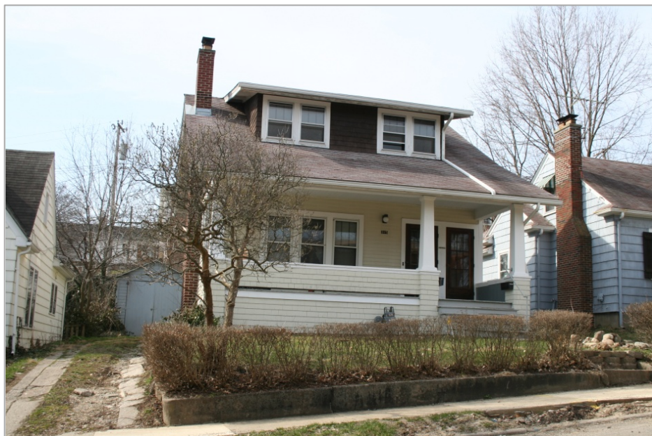
315 Koch Street (April 2008 survey photo)
